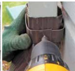
Wiggle the attached downspout assembly to make sure it is secure.
