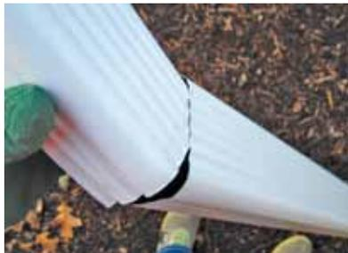
Attach extensions with two short sheet metal screws per joint. To prevent leaks, **do not put screws in the bottom** of any pieces.
