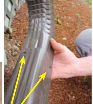
Place screws only on the top or side of the gutter.
