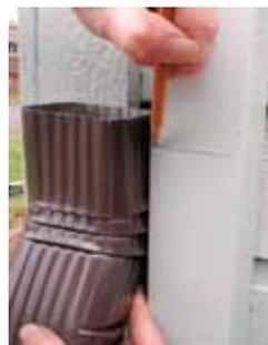
Mark the connected downspout one inch below where the elbow/extension assembly lines up with it. This is where you will cut.
