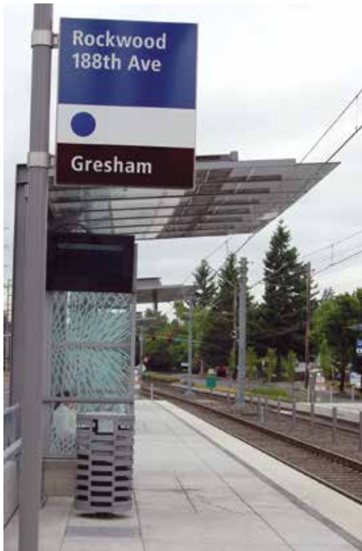
The Rockwood/E 188th Avenue MAX light rail station received major upgrades in 2011.
