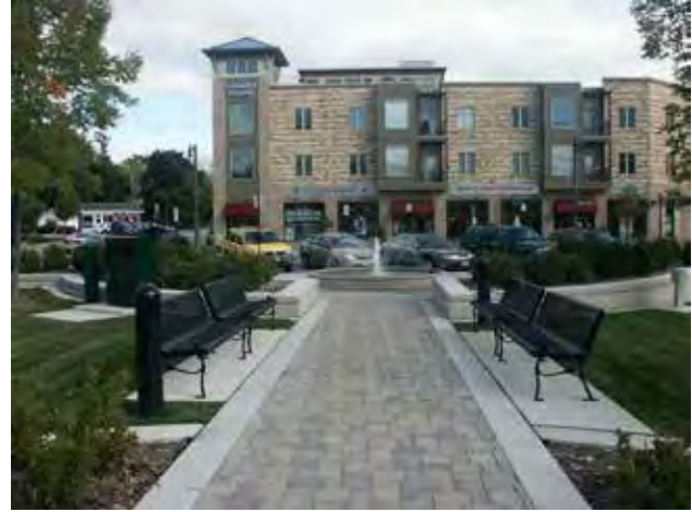
Fig. A.7.C.3.a: A walkway which connects an open space to an abutting mixed-use building.
