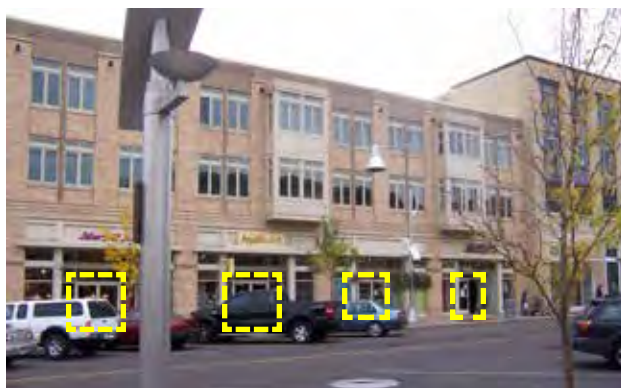
Fig. A.4.D.4: A multi-tenant building over 120 feet in length with multiple street-facing entries.
