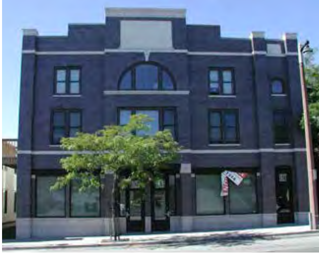
Fig B.5.D.2: A small projection, complimented by a taller parapet and unique windows, gives prominence to the entry.
