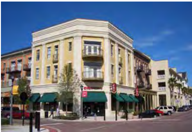
Fig B.6.D.2: Facade sections fronting the Gateway intersections shall be at least 3 occupiable stories.
