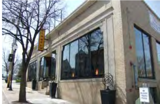
Fig B.4.C.3 OUTSIDE THE TRIANGLE: Facades facing the primary street of the site shall have the highest level of transparency.
