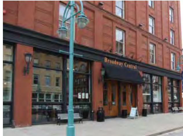
Fig B.3.C.1: The ground level is enhanced by features including light fixtures, an awning over the door and transom windows.
