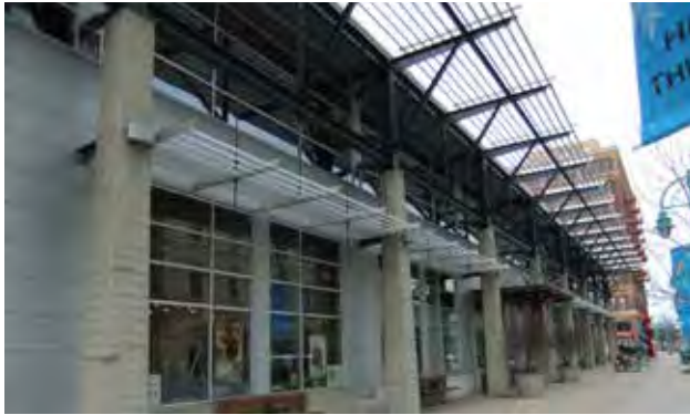
Fig C.1.D.4.b.iii: Solar shades are used to minimize summer heat gain while allowing passive heating in the winter.
