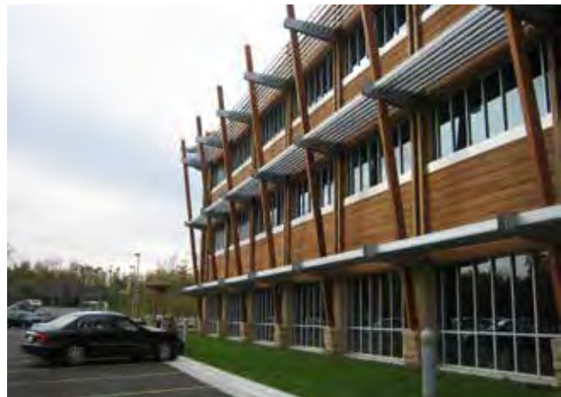
Fig B.4.C.4: Non-street facing facades shall include transparency to allow passive observation of the parking area.
