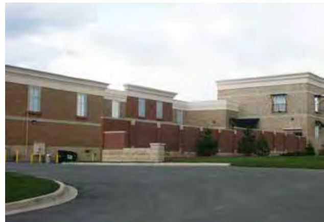
Fig. A.9.C.3: A service area is screened by walls with a character similar to the adjacent building.
