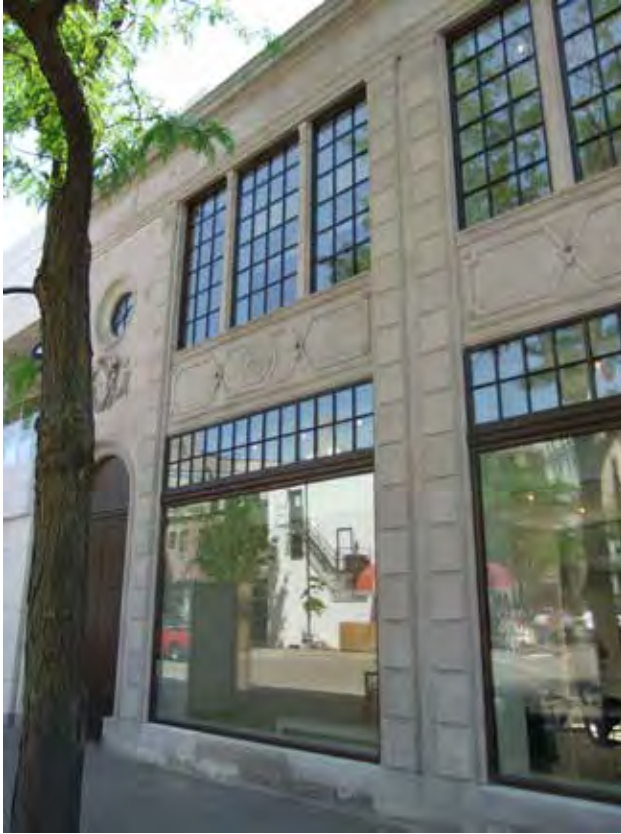
Fig B.4.D.5: The upper level incorporates vertically-oriented windows to increase transparency and prevent a dominant horizontal geometry in the facade.
