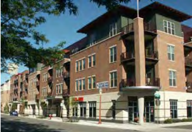
Fig B.3.D.3: A building base which utilizes a change in material. A full story base may be appropriate on taller multi-story buildings.
