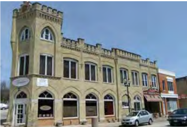
Fig B.2.D.4.e: In addition to changes in wall plane, pointed and round arches over windows enhance the facade.
