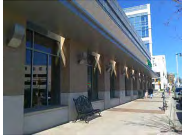
Fig. B.3.D.1.c and n: Projecting sills and wall-mounted lighting fixtures add detail to this commercial building's facade.
