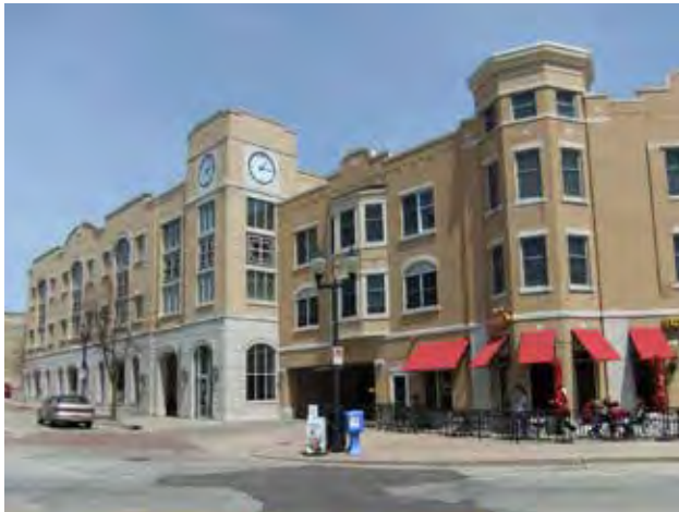
Fig B.1.D.2: Changes in building mass are visible from the street.
