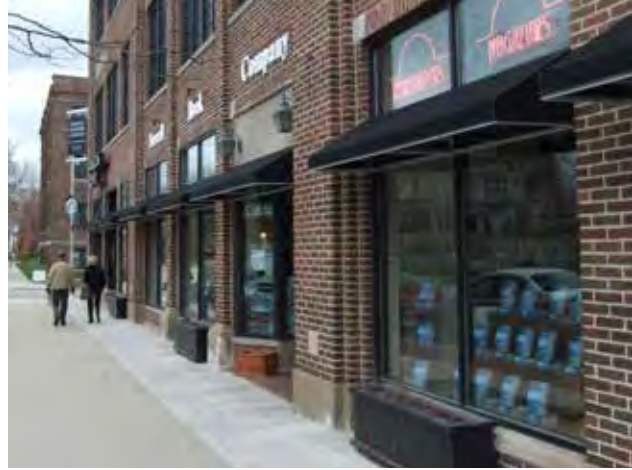
Fig B.4.C.1: Ground floor windows are recessed from the building wall to create depth.
