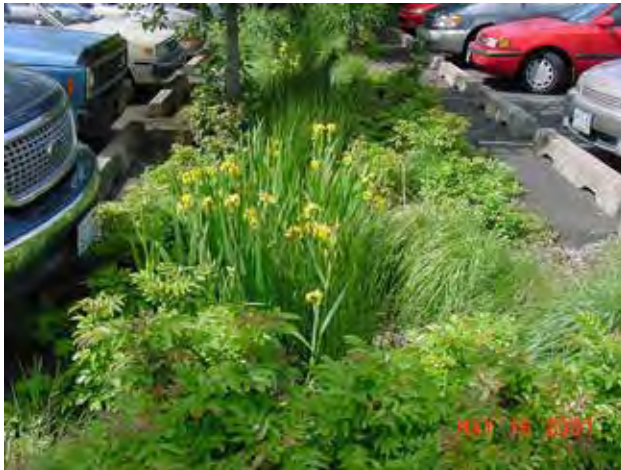
Fig. C.1.C.2(4): A stormwater swale within a parking lot filters and manages the pavement run-off.
