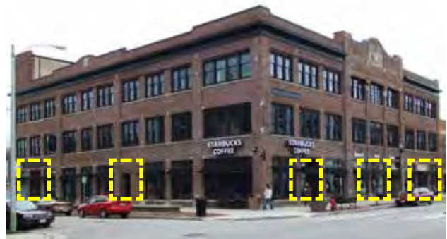
Fig. A.4.C.4: A mixed-use building with entries for each ground floor retail tenant and separate entrances for upper level uses.
