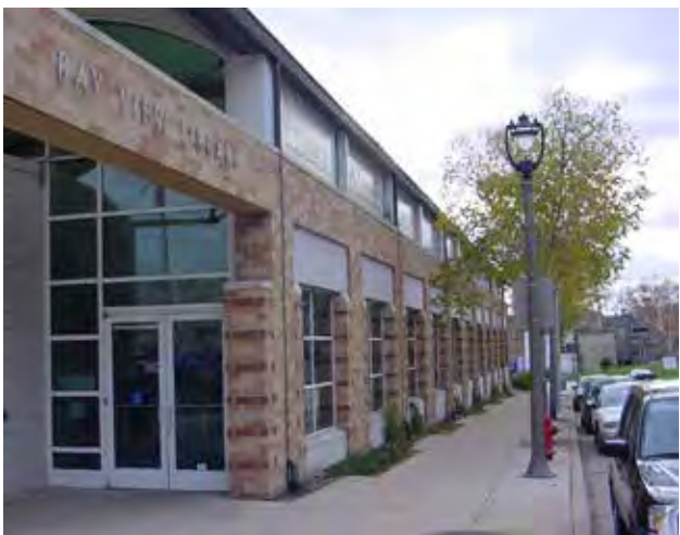
Fig. B.2.C.4: Recessed windows create depth in the facade.
