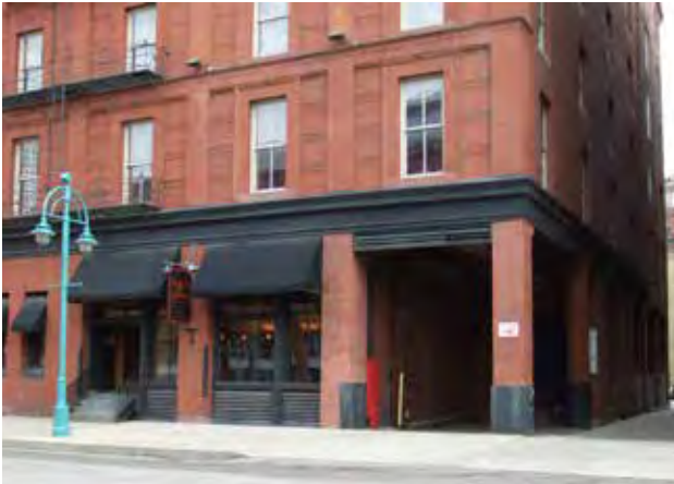
Fig. A.9.D.1(a): A loading area that is incorporated into the side of a building, but located away from the entry and other active areas.
