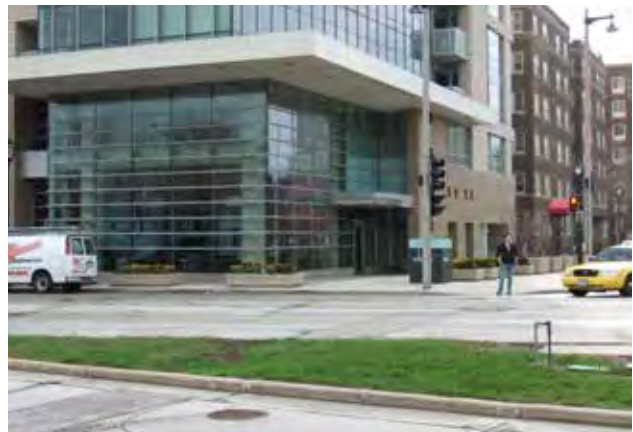
Fig B.4.D.9: Lobbies and other common areas shall have increased levels of transparency in multi-family buildings.
