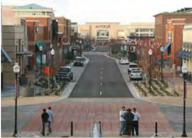
Fig. A.2.C.2(3): Pedestrian conflicts are minimized by limiting driveways and providing visually distinct crosswalks.
