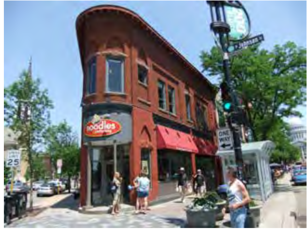
Fig B.6.D.4: High-quality materials, including brick, stone and glass, are used on facades facing important intersections.
