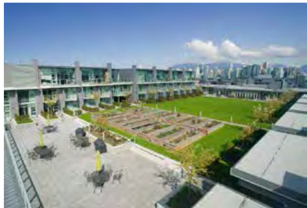
Fig C.1.D.4.b.ii(3): A large green roof reduces heat islands, minimizes stormwater and provides residents with a roof-top amenity in this mixed-use development.
