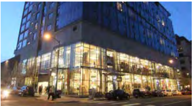
Fig. A.10.D.1: Storefronts and exterior light fixtures create uniform illumination levels at the building entry.
