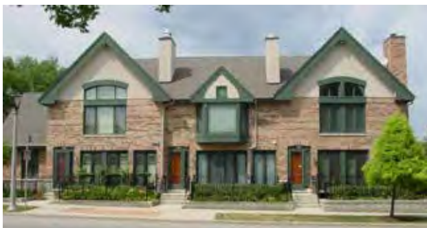
Fig. A.4.D.9(d): Landscaping behind a decorative metal fence defines private space at the street edge.
