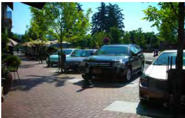
Fig C.1.D.2.e: Permeable pavement allows water to infiltrate the soil thereby reducing stormwater discharge.
