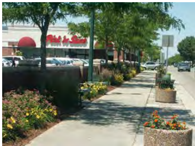
Fig. A.6.D.7 OUTSIDE THE TRIANGLE: A limited amount of parking may be placed on the side of a building at the street edge when screening is present.
