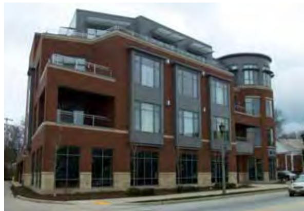
Fig. B.2.C.4 OUTSIDE THE TRIANGLE: Changes in wall plane are used to create visual interest and reduce the perceived scale of wall planes.
