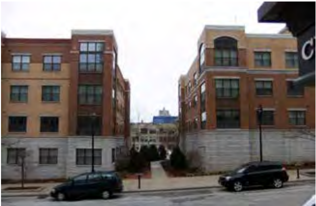
Fig. A.6.C.3: A defined walkway links the parking area to the street and sidewalk.
