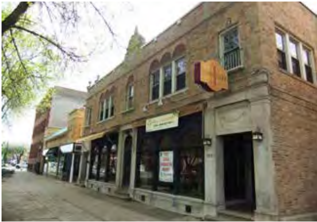
Fig B.5.D.3.b: A change of materials highlights the entries to this traditional storefront.
