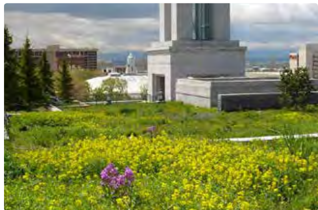
Fig C.1.C.2(3): This green roof provides an attractive, sustainable habitat for wildlife.
