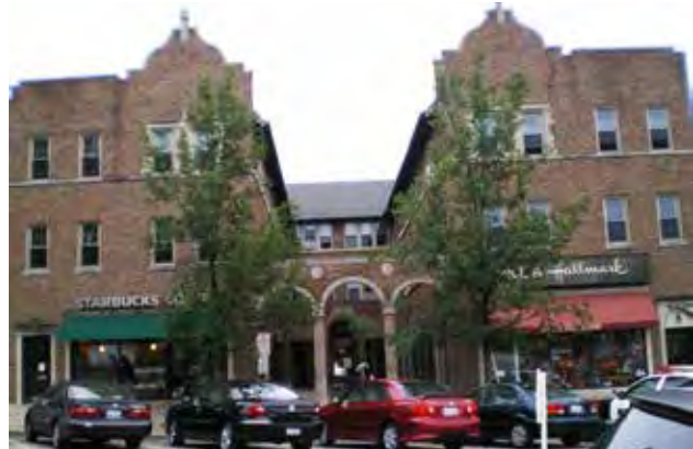
Fig B.5.C.2: An entry courtyard is used to distinguish it from the rest of the facade.
