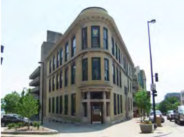
Fig B.4.D.11: A renovated building in which windows were reinstalled.
