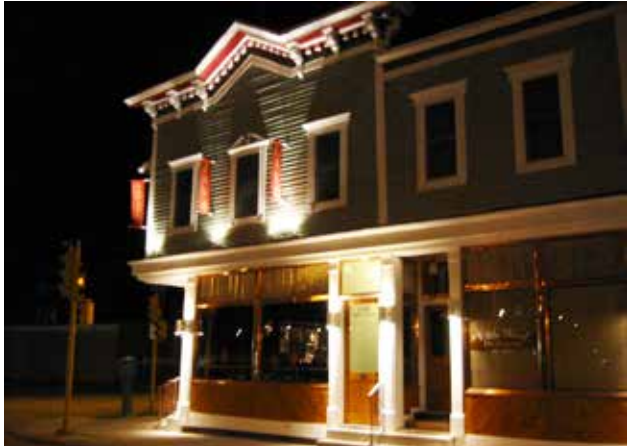
Fig. A.10.C.7: Light fixtures can highlight architectural features but caution should be used to prevent sky-glow.
