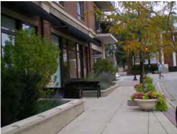
Fig B.3.D.4: Integrated planters may be used in place of a building base.
