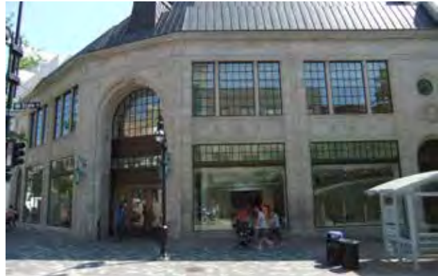
Fig B.5.C.1: Building entries shall be a prominent element in the facade.
