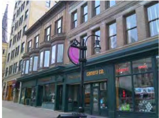
Fig. A.4.C.1: A building oriented toward the street with entries present on the sidewalk.
