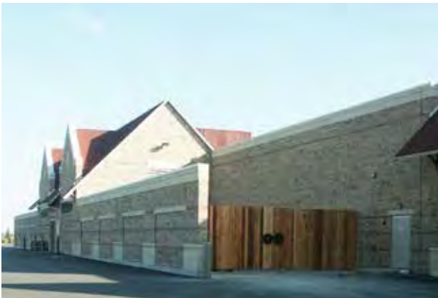
Fig. A.9.D.1(b): Screening wall of a loading area using similar materials and articulation as the primary structure.
