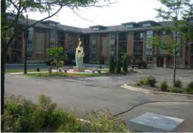
Fig. A.8.D.5: An attractively landscaped parking area of a multi-family building includes trees, shrubs and a sculpture.
