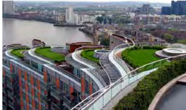
Fig C.1.D.4.b.ii(2): These green roof gardens help purify the urban air and lower urban air temperatures.
