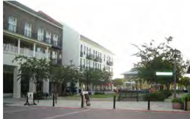
Fig. A.5.C.4: A public space adjacent to the street and at the same grade ensures physical and visual connection to the street and accessibility of all users.
