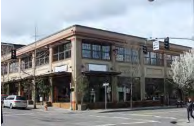
Fig B.2.D.4.a: A building which is designed with pilasters and belt courses to enhance the facades.
