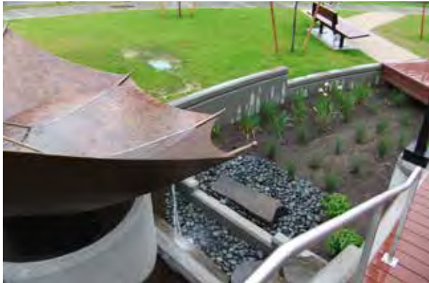
Fig C.1.D.2.c: A public art piece collects rain water and discharges it into a stormwater area.
