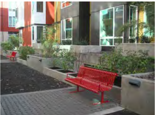
Fig. A.5.D.5(f): A pedestrian space incorporates pervious paving and other stormwater management techniques.
