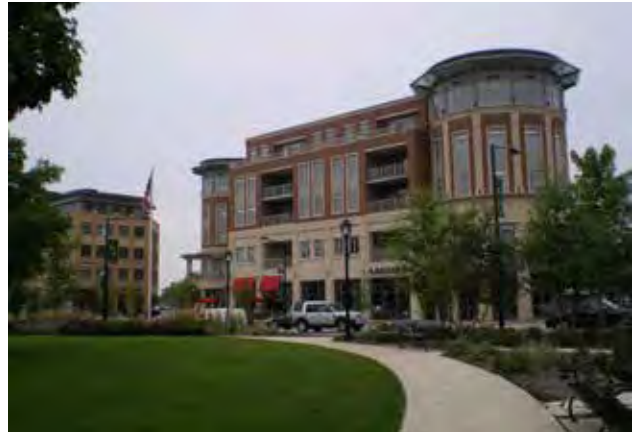
Fig B.1.C.5: Changes in building massing frame the public space and highlight important locations, such as street intersections.
