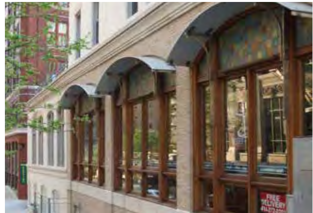
Fig B.7.C.1(2): A brick storefront enhanced with ceramic tiles highlighting the windows.
