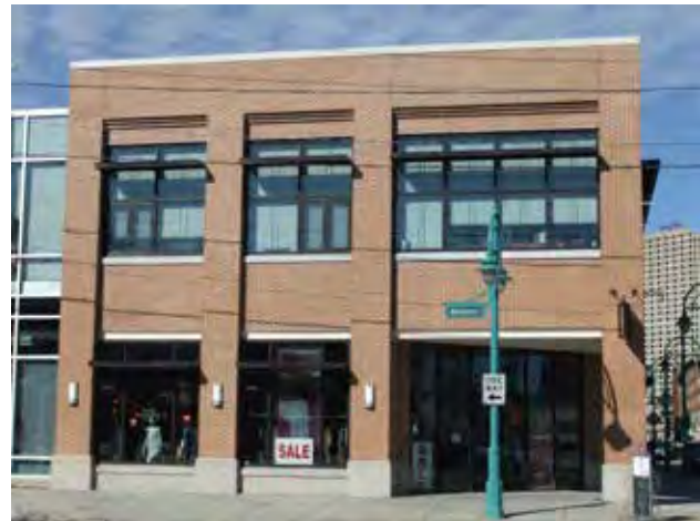
Fig B.3.C.3: A defined base transitions the building facade to the ground and complements other features on the building.
