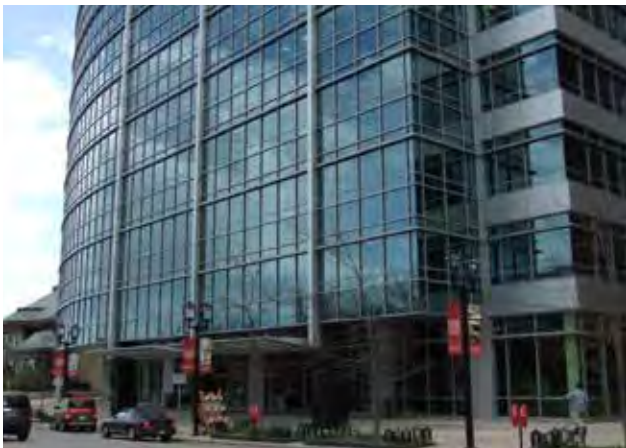
Fig B.2.D.4.b: Major vertical mullions, in conjunction with a change in plane, visually break up an all glass facade.
