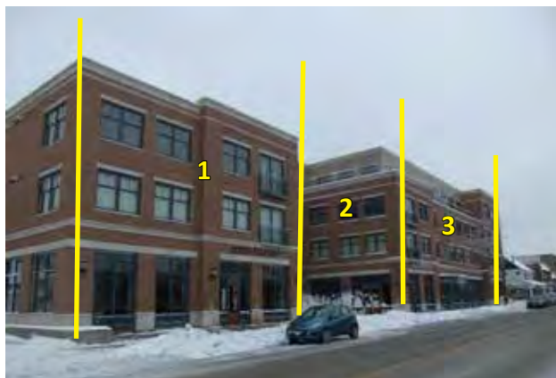
Fig B.1.D.3: A building with a large footprint is divided into multiple masses, each greater than 25% of the footprint.
