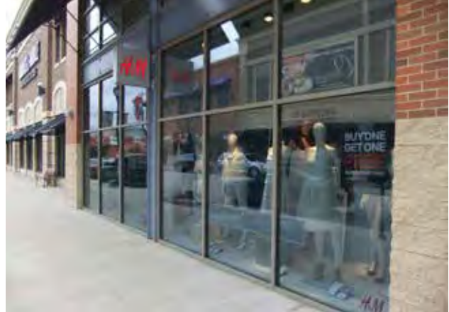
Fig B.4.D.7: A limited amount of displays which extend into the building may count toward the transparency requirement.
