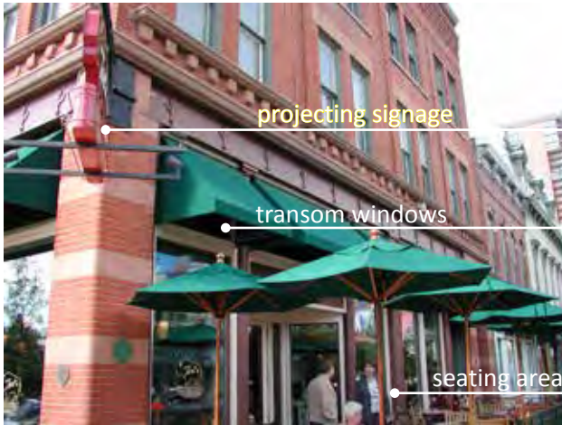
Fig B.3.D.1.b, h, i, m, s and t: Transom windows, projecting signage and a seating area enhance the facade's ground level.
