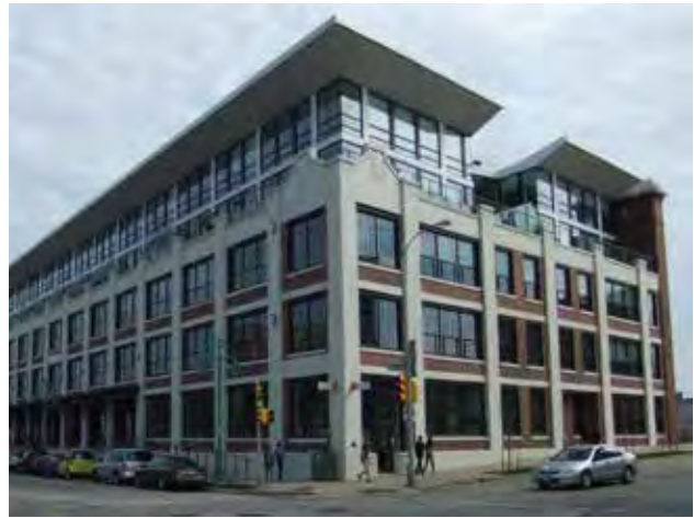
Fig B.1.D.9: An addition (above the original three stories) to a historic building that is visually distinct and complementary to the original form.
