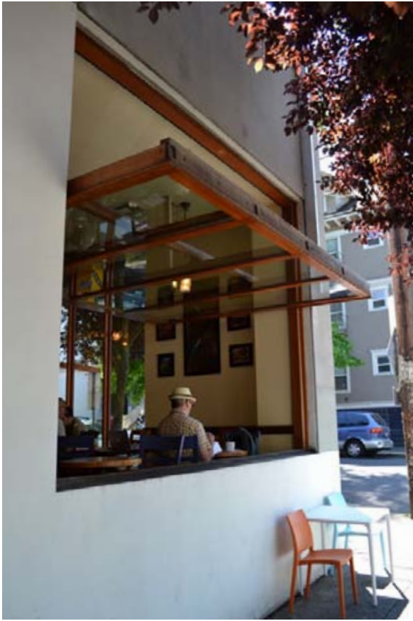
A display window converted to a large pivot window
