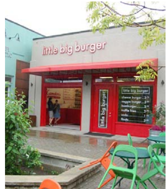
Bold Color and operable storefront make for an inviting entry.
