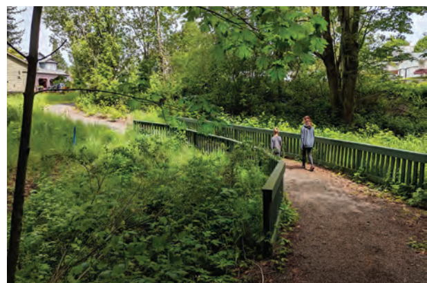
Kelly Creek Tributary Footbridge
