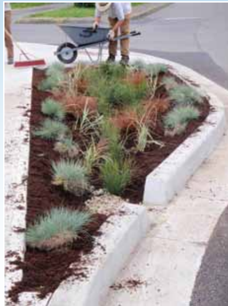
Installing a rain garden at the Center for the Arts Plaza.
