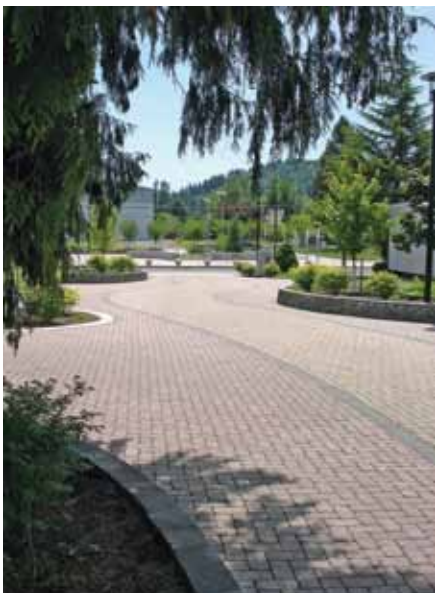
Beech Street, Gresham's first green street, wins National American Public Works Association award for its innovative design to minimize impacts to the environment.
