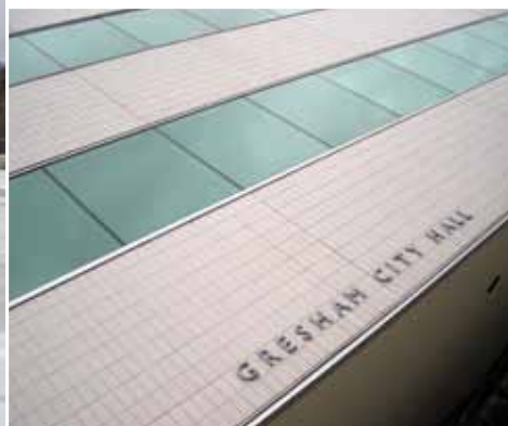
Left: City Hall's white roof reflects the hot sun, helping keep internal temperatures down. Skylights light three flights of stairs in two stairwells inside City Hall.
