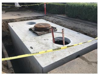
Tanks and vaults require a sedimentation manhole to capture sediment upstream of the tank or vault. The sedimentation manhole does not provide adequate water quality treatment, so a stormwater quality treatment facility is required to meet pollution reduction requirements. The vegetated facilities listed in **section 3.2** are considered to be adequate pre-treatment by the City, but a proprietary device may be proposed if infeasibility has been demonstrated per **section 1.2.2**.
