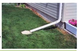
Site conditions will determine if this is a suitable method for managing stormwater onsite. Property line and building setbacks as well as surface grade and available landscaped areas for infiltration must be considered. Proposed downspout locations and roof/gutter alignments will impact the feasibility of this option. As such, a preliminary site visit by City staff is recommended to determine if downspout extensions are a viable option.
