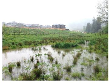
meet water quality and detention requirements require plantings around the perimeter of the pond (within an aquatic bench) following the requirements in **Appendix G**.
