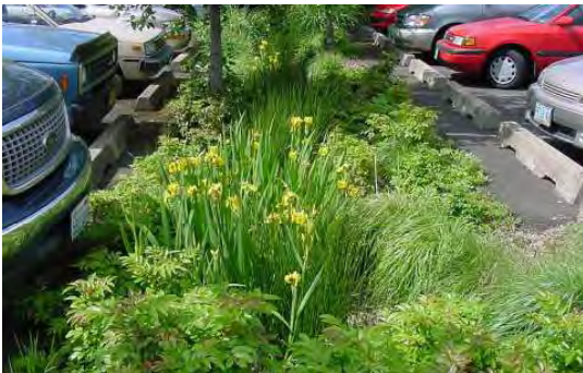
Fig. A.6.S3.a: A stormwater swale within a parking lot filters and manages the pavement run-off.
