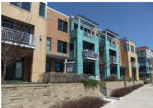
Fig B.4.S11: An elevated landscaped area and a decorative wall create a division between public and private space.
