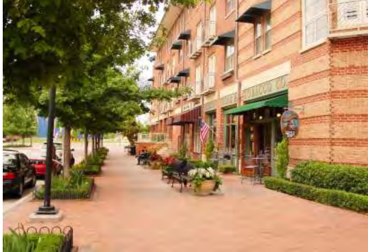
Fig. A.5.S6.b: Sidewalks that received additional design features may be counted as pedestrian-oriented open spaces.
