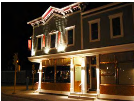
Fig. A.7.G2: Light fixtures can highlight architectural features but caution should be used to prevent sky-glow.
