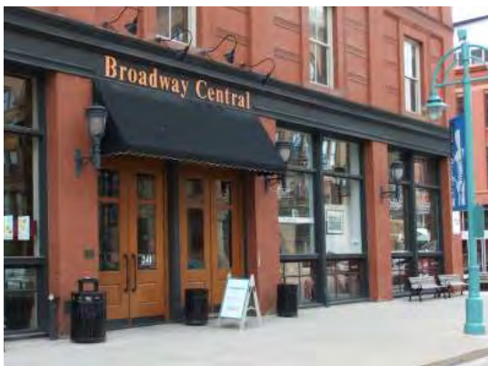
Fig B.3.G7: Areas surrounding the entry shall utilize high-quality materials such as brick.
