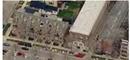
Fig. B.2.S1: A flat roof is painted white for a high SRI value.
