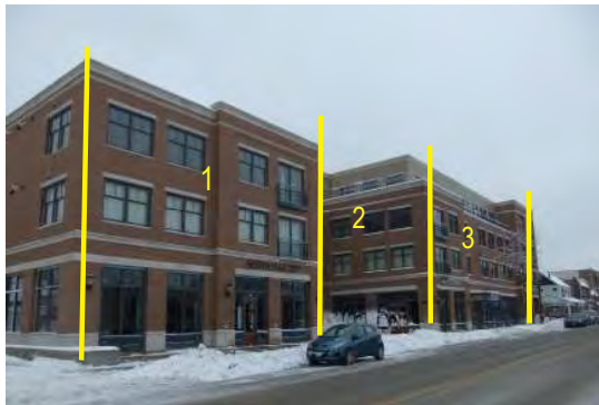
Fig B.1.S8: A building with a large footprint is divided into multiple masses, each greater than 25% of the footprint.
