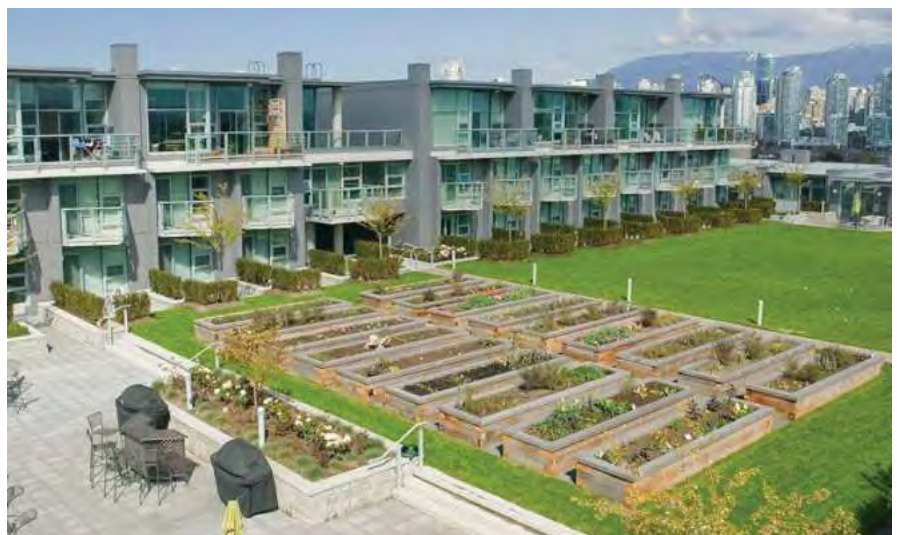
Fig B.4.S3.f: A large green roof reduces heat islands, minimizes stormwater and provides residents with a roof-top amenity in this mixed-use development.
