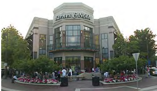
Fig B.6.S5: Landscaped plazas with pedestrian amenities encourage activity at the Gateways.
