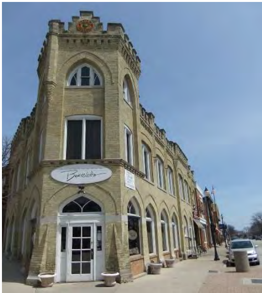
Fig B.1.S5.a: A tower form on a building fronting a major intersection adds prominence to the location.
