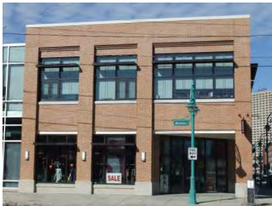
Fig B.4.G7: A defined base transitions the building facade to the ground and complements other features on the building.
