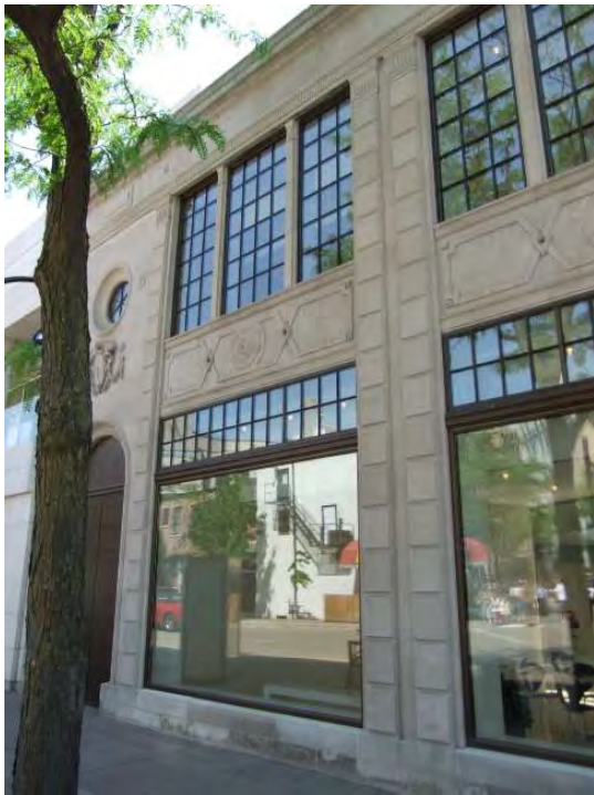
Fig B.5.S5 and B.5.S6.a: The upper level incorporates vertically-oriented windows to increase transparency and prevent a dominant horizontal geometry in the facade.
