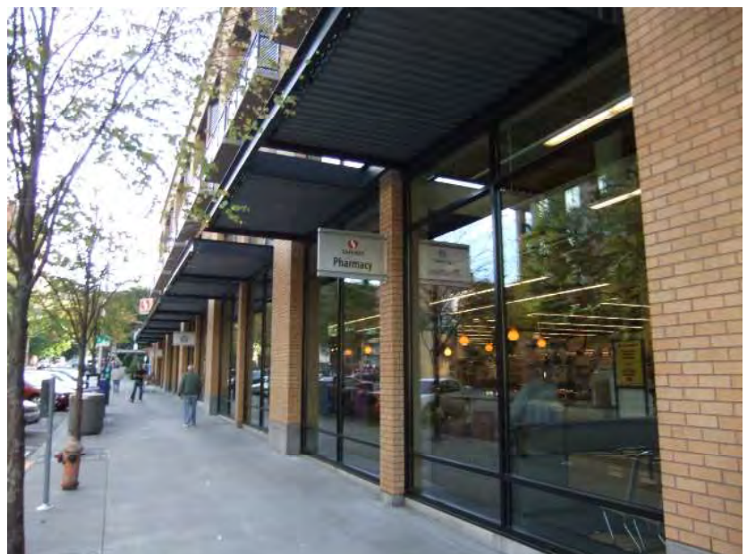
Fig B.5.S1: Storefront windows recessed to establish depth.
