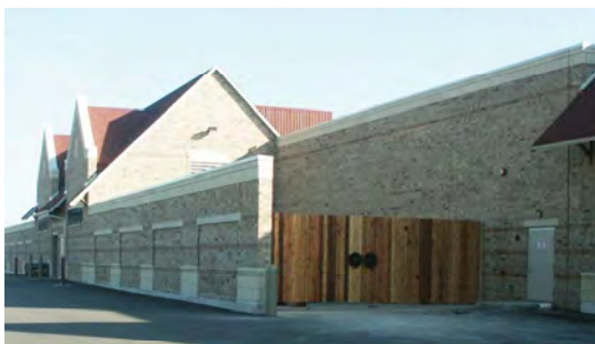
Fig. A.4.S6.b: Screening wall of a loading area using similar materials and articulation as the primary structure.
