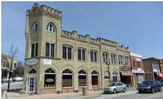
Fig B.4.S4: In addition to changes in wall plane, pointed and round arches over windows enhance the facade.
