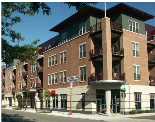
Fig B.4.S7: A building base which utilizes a change in material. A full story base may be appropriate on taller multi-story buildings.
