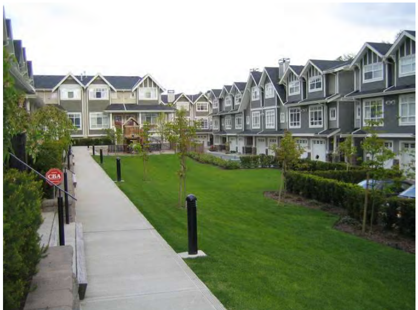
Fig. A.5.S7: A shared open space which is fronted by several multifamily buildings.
