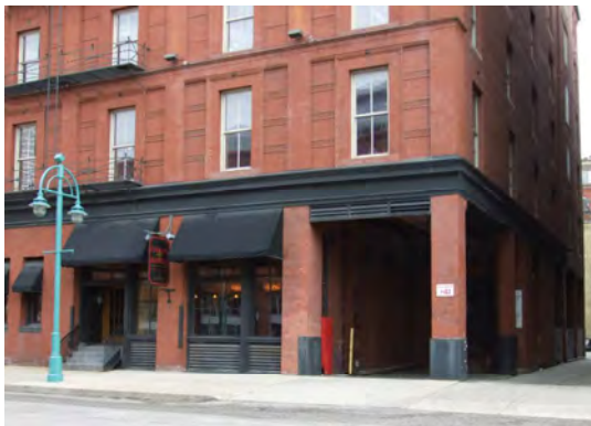
Fig. A.4.S6.a: A loading area that is incorporated into the side of a building, but located away from the entry and other active areas.
