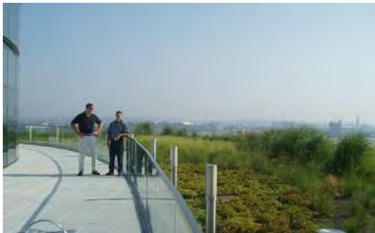
Fig B.4.S3.b: This Hydrotech™ roof-top garden provides attractive functional open space while saving building energy costs.
