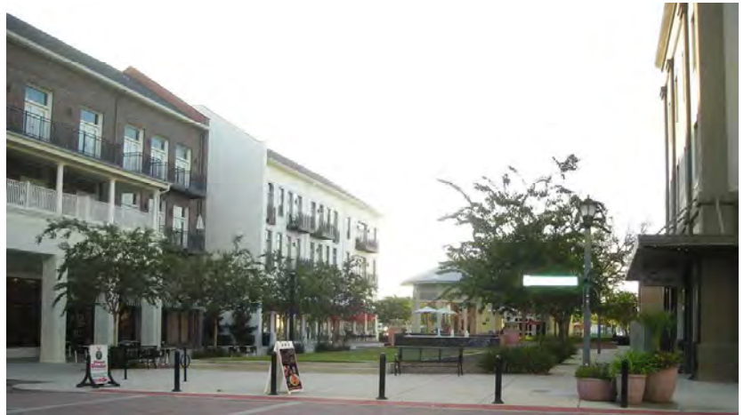
Fig. A.5.G4: A public space adjacent to the street and at the same grade ensures physical and visual connection to the street and accessibility of all users.
