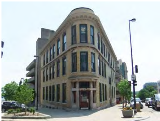
Fig B.5.S11: A renovated building in which windows were reinstalled.
