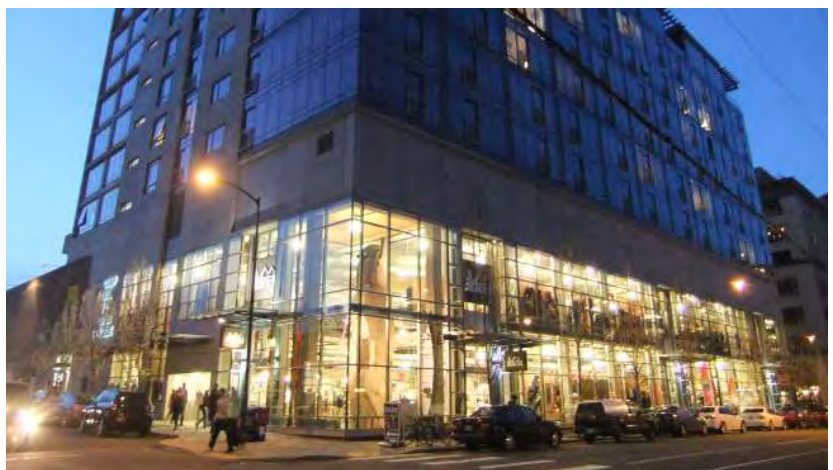
Fig. A.7.S1: Storefronts and exterior light fixtures create uniform illumination levels at the building entry.
