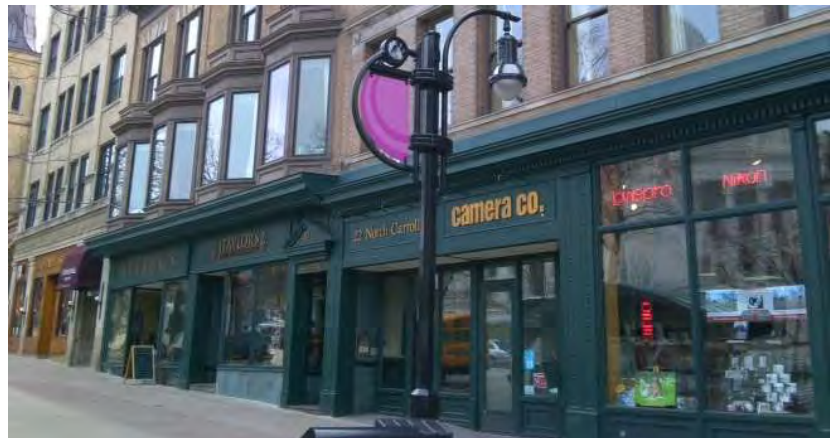
Fig. B.3.G1: A building oriented toward the street with entries present on the sidewalk.
