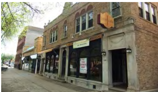
Fig B.3.S6: A change of materials highlights the entries to this traditional storefront.
