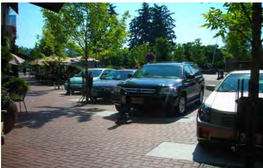
Fig A.6.S3.c: Permeable pavement allows water to infiltrate the soil thereby reducing stormwater discharge.
