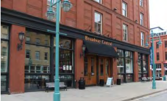
Fig B.4.G5: The ground level is enhanced by features including light fixtures, an awning over the door and transom windows.
