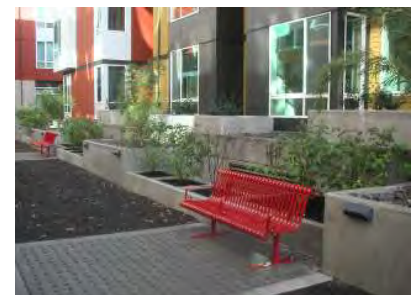
Fig. A.5.S5.b: A pedestrian space incorporates pervious paving and other stormwater management techniques.
