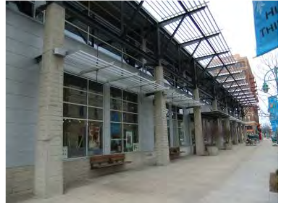
Fig B.4.S3.a: Solar shades are used to minimize summer heat gain while allowing passive heating in the winter.
