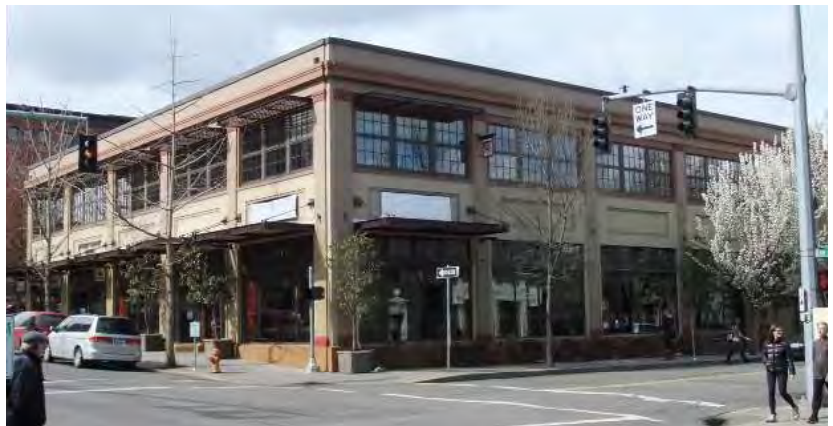
Fig B.1.S12: A building which is designed with pilasters and belt courses to enhance the facades.
