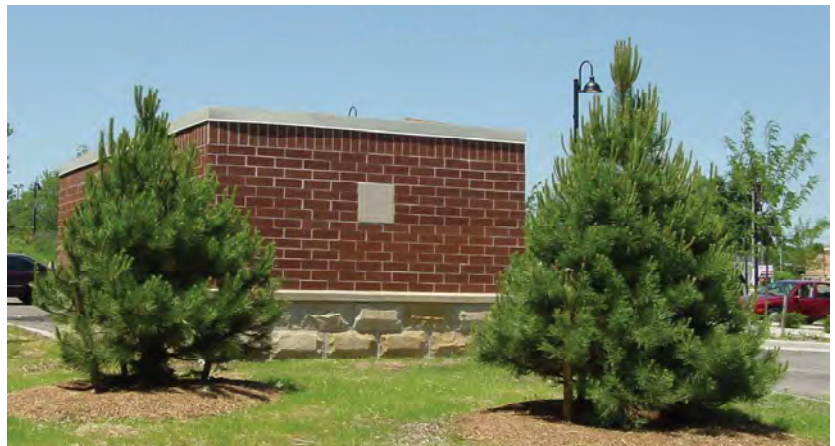
Fig. A.4.S7: A masonry enclosure screens dumpsters while complimenting the design of the building.
