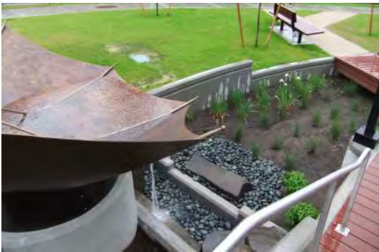
Fig A.6.S3.b: A public art piece collects rain water and discharges it into a stormwater area.
