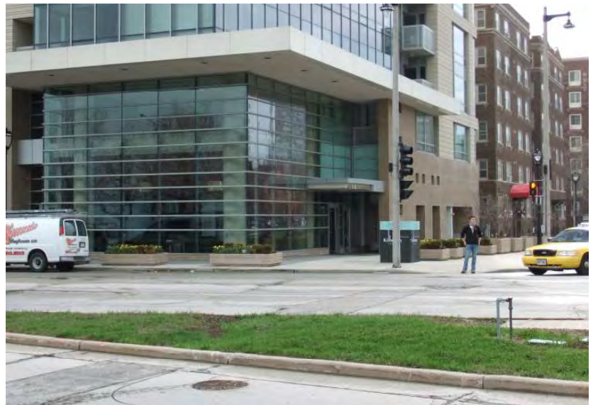
Fig B.5.S9: Lobbies and other common areas shall have increased levels of transparency in multifamily buildings.
