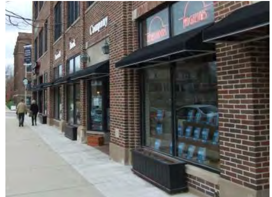
Fig B.5.G1: Ground floor windows are recessed from the building wall to create depth.
