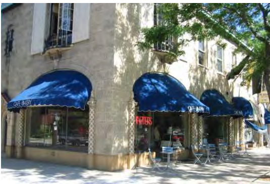
Fig B.4.S5.d: Large awnings shade windows and provide weather protection on the ground level of a commercial building.
