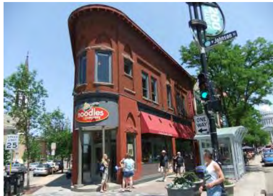
Fig B.6.S4: High-quality materials, including brick, stone and glass, are used on facades facing important intersections.
