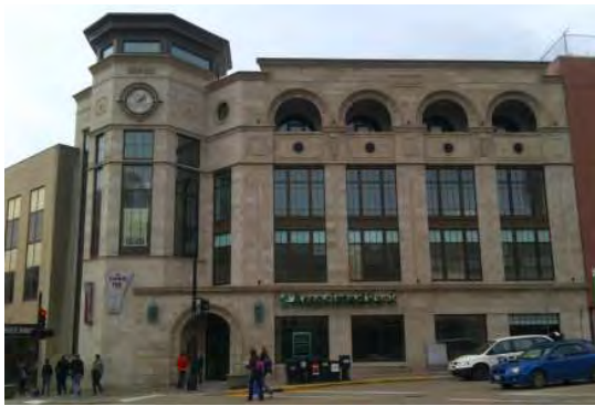
Fig B.6.G4.a: Stone and other high-quality materials are appropriate for highly visible gateway buildings.
