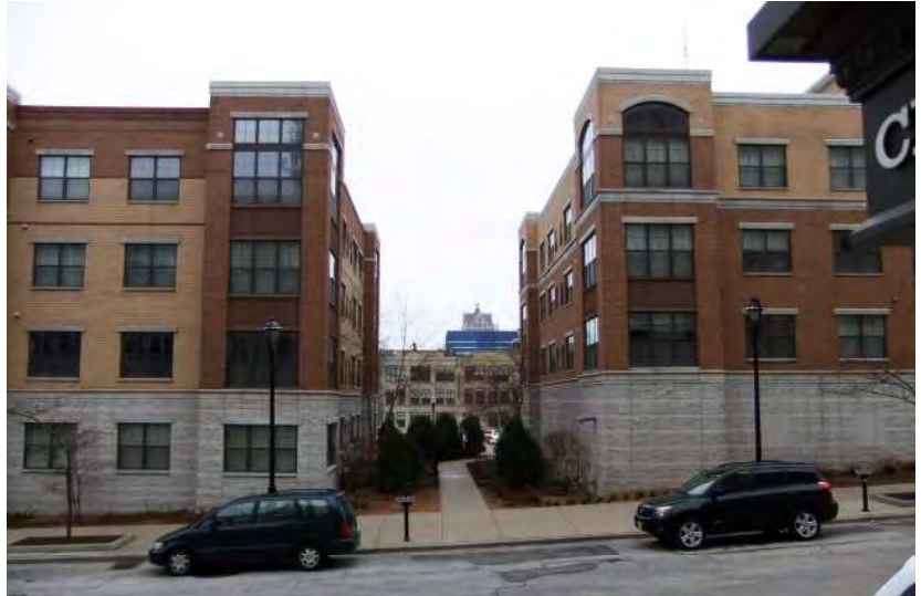
Fig. A.3.S3: A defined walkway links the parking area to the street and sidewalk.
