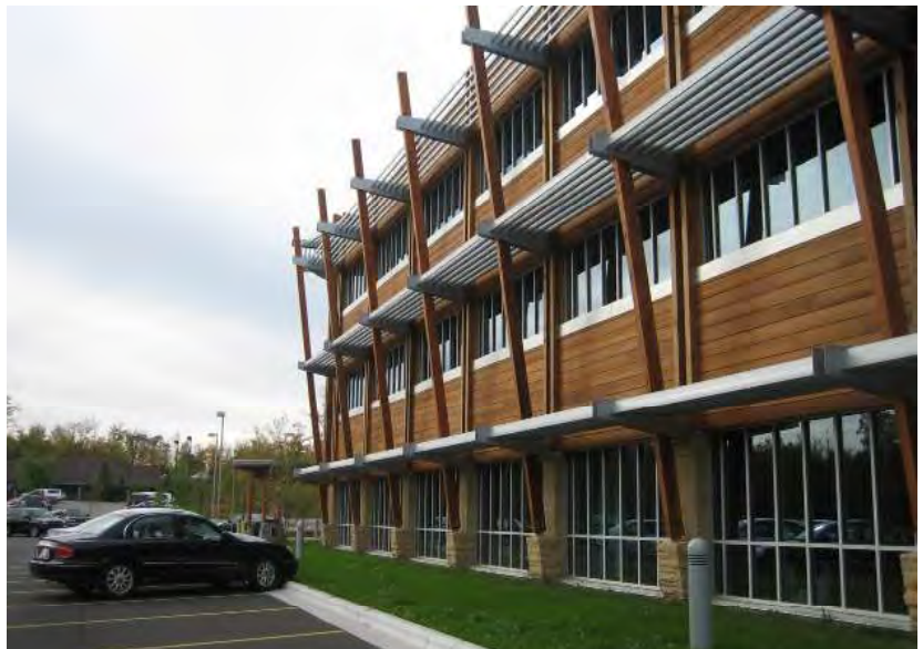
Fig B.5.G4: Non-street facing facades shall include transparency to allow passive observation of the parking area.
