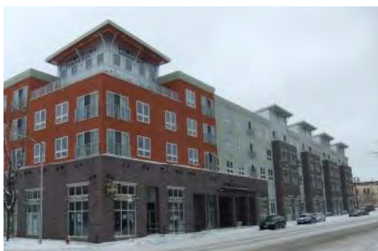
Fig B.6.G3: Building entries shall be very close to gateway intersections to encourage pedestrian activity in these areas.
