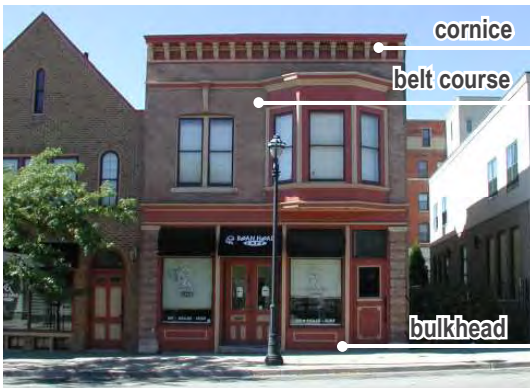
Fig B.1.G12.a INSIDE THE TRIANGLE: Horizontal elements, including a series of belt courses, the cornice and the bulkhead, establish rhythm in the storefront.
