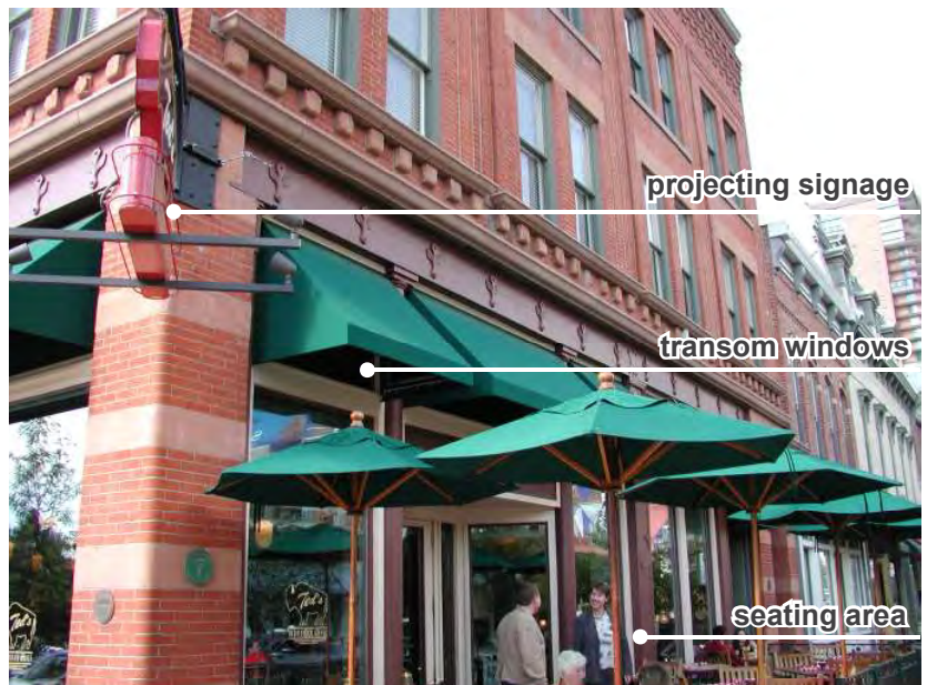
Fig B.4.S5.e: Transom windows, projecting signage and a seating area enhance the facade's ground level.
