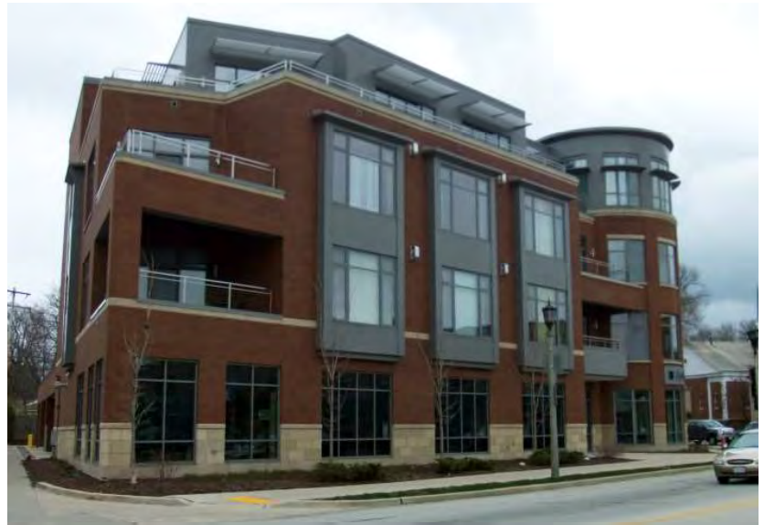
Fig. B.1.G12.b OUTSIDE THE TRIANGLE: Changes in wall plane are used to create visual interest and reduce the perceived scale of wall planes.
