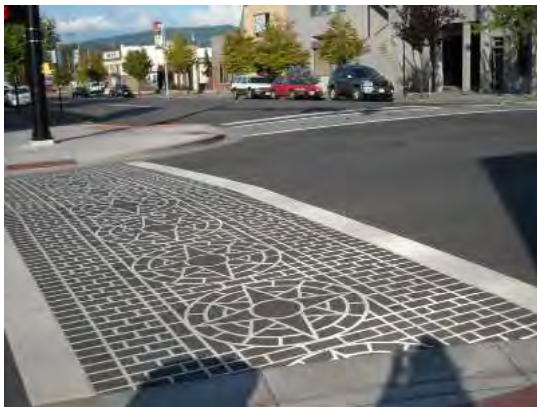
Fig. A.1.S7: Bump-outs and crosswalks with decorative paving are present on primary internal drives when parking is included.
