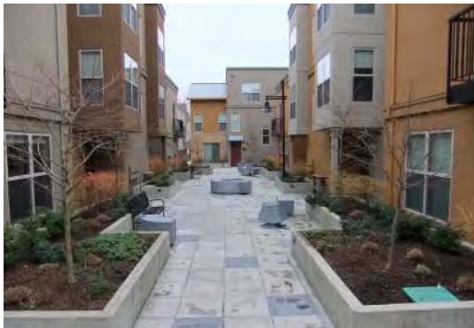
Fig. A.3.G4: A walkway provides additional connectivity where an automobile connection would not be feasible.
