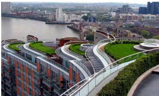
Fig B.4.S3.c: These green roof gardens help purify the urban air and lower urban air temperatures.
