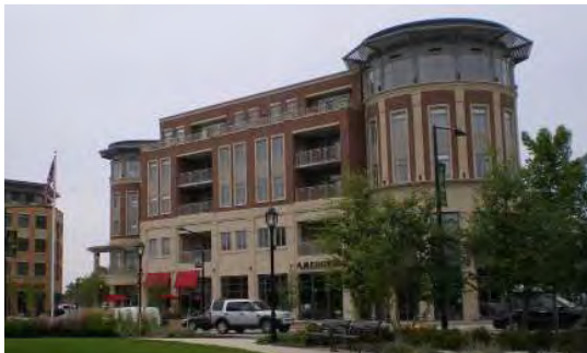
Fig B.1.G10: Changes in building massing frame the public space and highlight important locations, such as street intersections.
