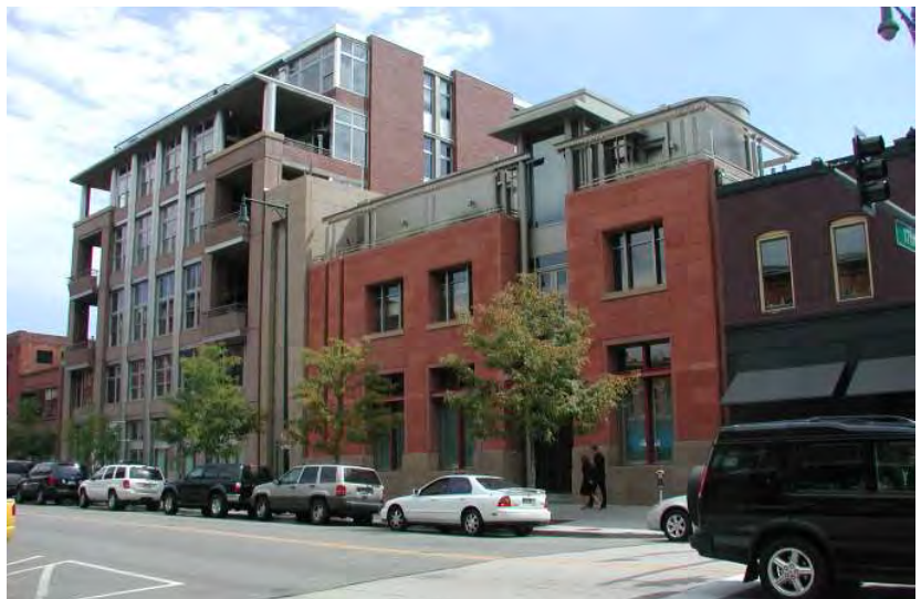
Fig B.1.G9: Changes in massing create depth in the facade and are sufficient to provide visual distinction between wall planes.
