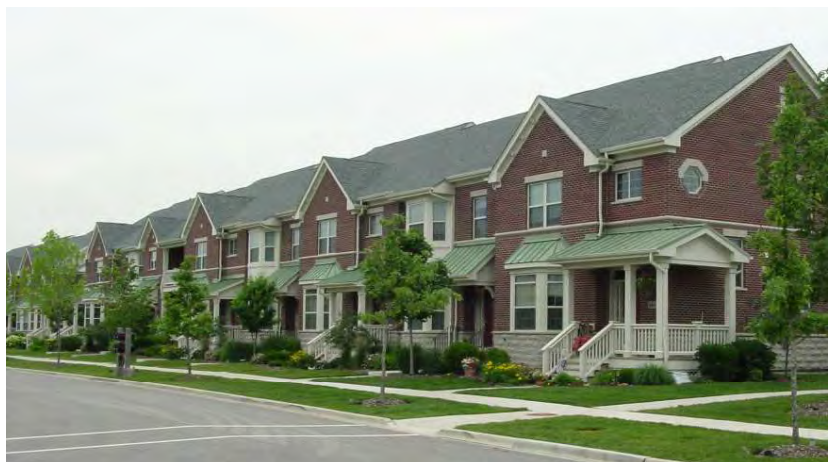
Fig A.2.S3 OUTSIDE THE TRIANGLE: Multifamily buildings shall be placed close to the street, but shallow setbacks are allowed to increase the level of privacy for individual units.
