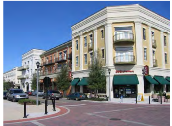
Fig. B.3: A commercial building with an entry located at the corner.
