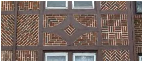
Fig B.4.S5.a: An example of ornamental brickwork in a mixed-use building.
