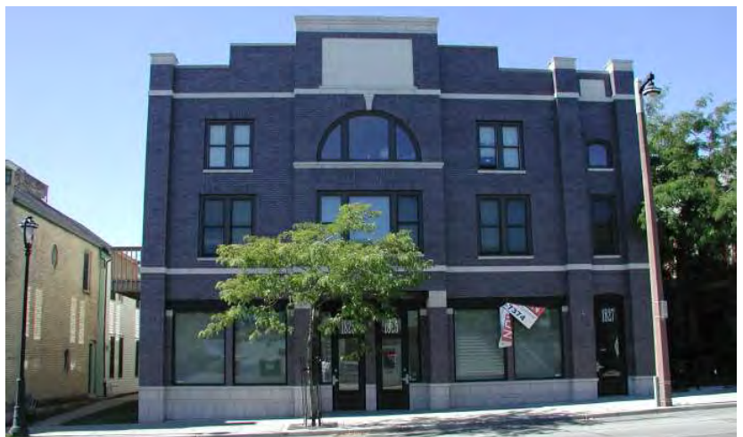
Fig B.3.S5: A small projection, complimented by a taller parapet and unique windows, gives prominence to the entry.
