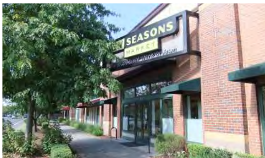
Fig A.2.S1 OUTSIDE THE TRIANGLE: Commercial buildings shall be placed close to the street with a landscaped area between the building and the sidewalk.
