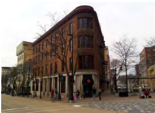
Fig. B.3.G2: A corner entry on a building located at the intersection of two streets.
