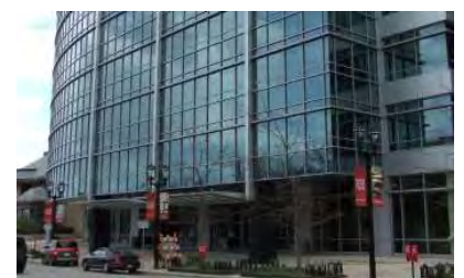
Fig B.1.S12.b: Major vertical mullions, in conjunction with a change in plane, visually break up an all glass facade.
