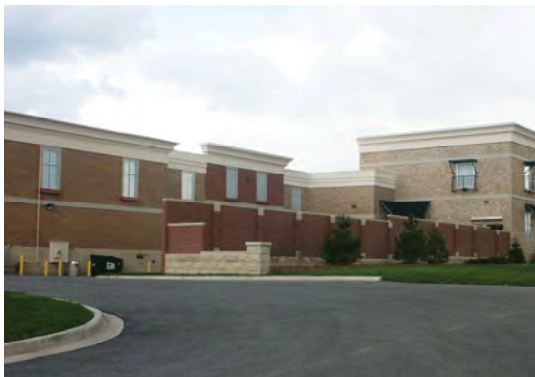
Fig. A.4.G8: A service area is screened by walls with a character similar to the adjacent building.
