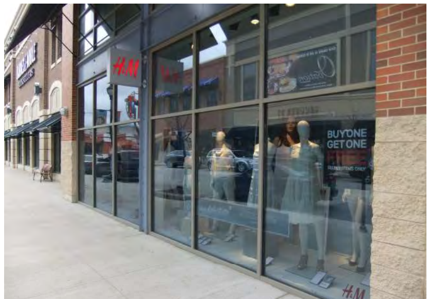
Fig B.5.S7: A limited amount of displays which extend into the building may count toward the transparency requirement.
