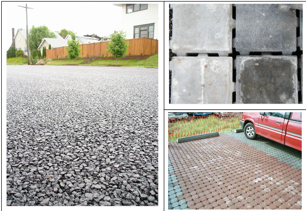
Left: porous asphalt mix. Top-right: SF RIMA™ pavers. Bottom-right: Uni Eco-Stone® pavers
