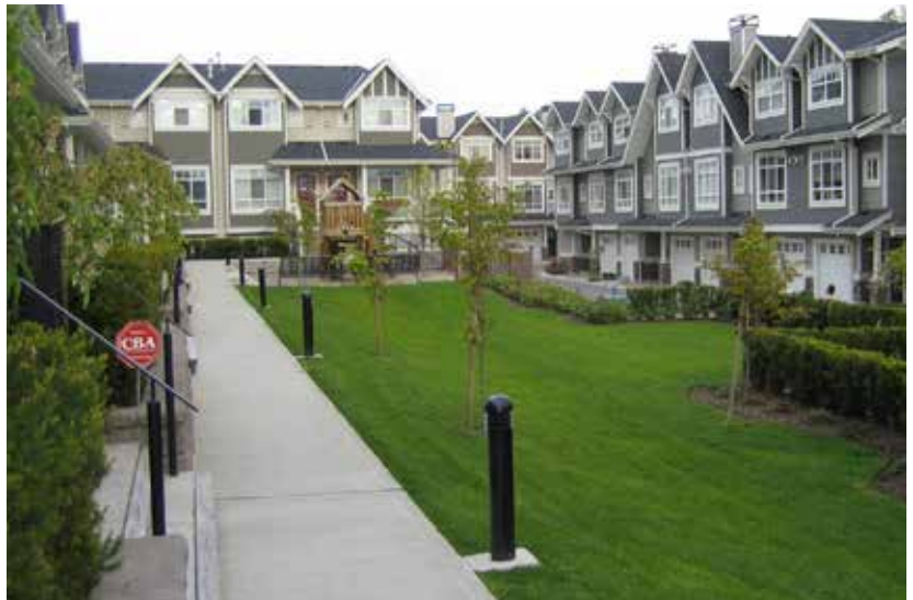
Fig. A.7.S3. Pedestrian-scaled bollard lighting with weather resistant coverings are located to illuminate a pedestrian walkway.
