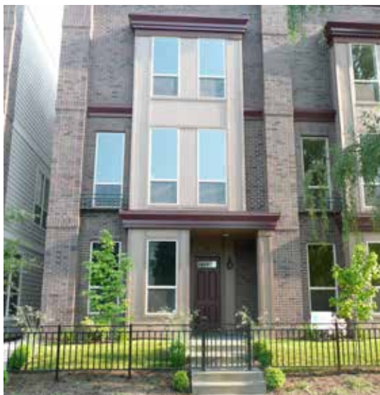
Fig. B.3.S5.b: Individual unit entry is framed by a wall recess and column.
