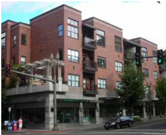
Fig. B.4.S5: A building base is established with a change in materials and fenestration pattern on the ground floor.
