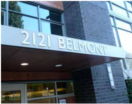
Fig. A.3.S4: Building address is illuminated and clearly visible.
