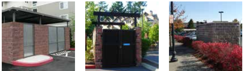
Fig. A.4.S5: Collection areas enclosed with walls using high quality building materials.
