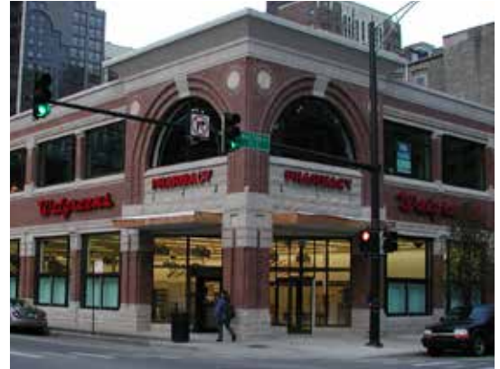
Fig. B.3: Recessed corner entry provides weather protection and access from both street frontages.
