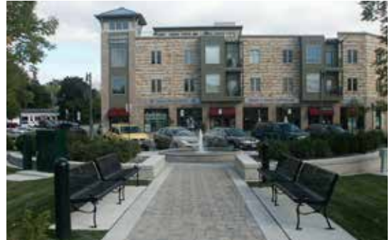
Fig. A.3: Pedestrian circulation route provides connections on and through the site.
