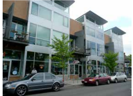
Fig. B.4: A repeating pattern of recesses and changes in wall planes create a pleasant rhythm in the facade which creates visual interest.
