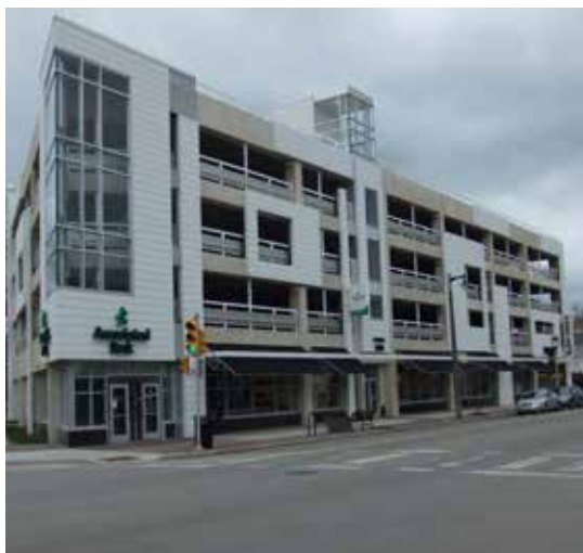
Fig. B.5.S2: Screening elements are used along the street facing facade of a large parking structure.
