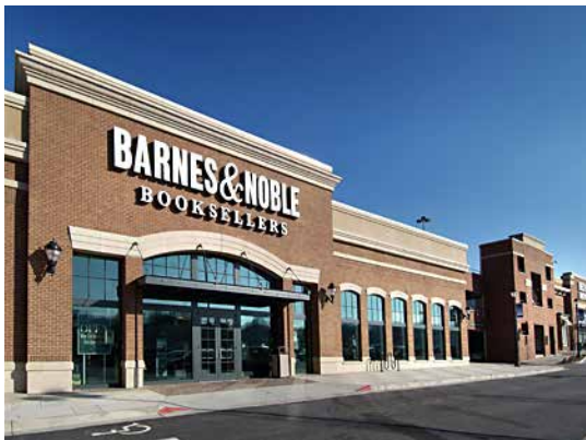
Fig. B.3.S3: The entry for the commercial building is highlighted with a visible change in the building form from adjacent facade sections, a change in the roof line, ornamental light fixtures, and oversize doors.
