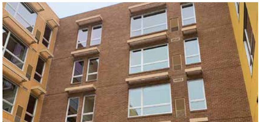
Fig. B.6.S1.a: A mixed-use building uses brick and glass as primary materials with fiber cement panels used as a secondary material.
