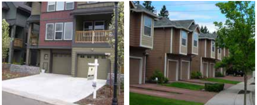
Fig. A.6.S15: Where driveways are not ganged together (left), a landscape strip separates driveways (right), allowing for rainwater infiltration opportunities and a softening of the street edge.
