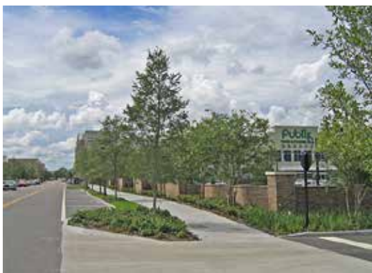
Fig. A.6.S5: Parking lot perimeter screening using a masonry wall with layered landscaping.
