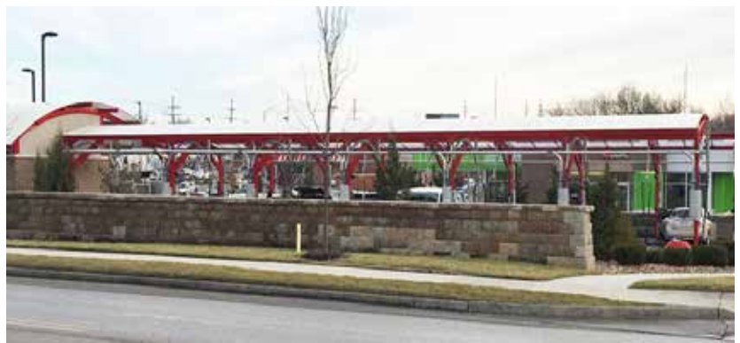
Fig. A.2.S4: For auto-dependent uses, alternative features such as a canopy with a decorative masonry wall may count toward the frontage requirement.
