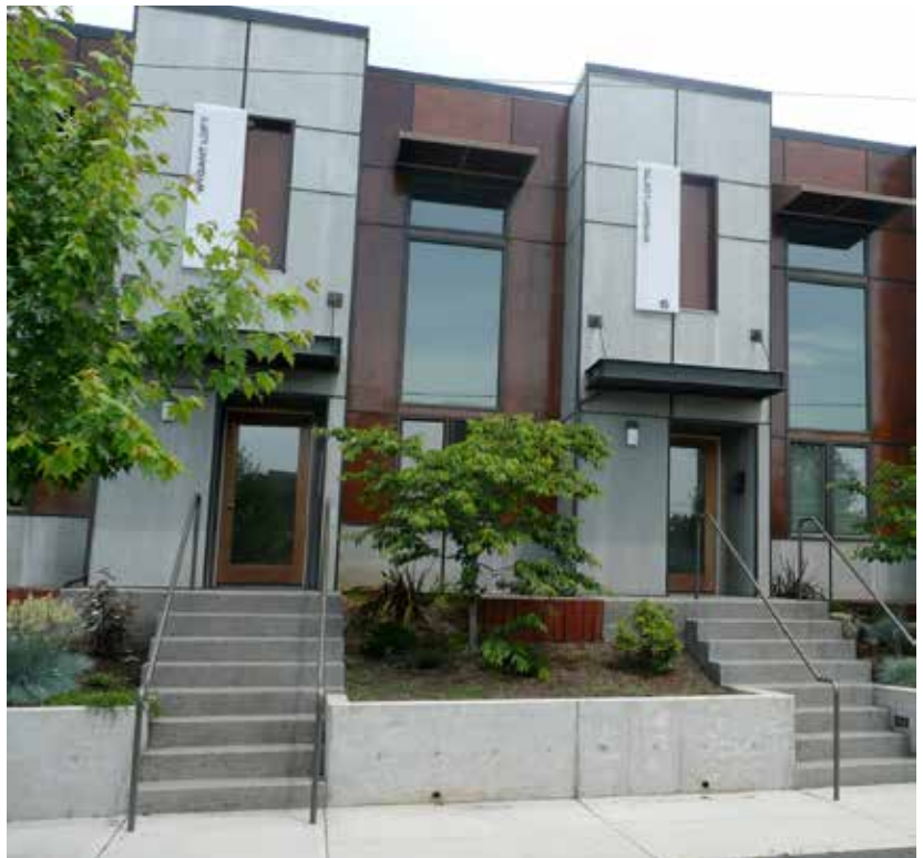
Fig. B.3.S9.d: A transition between the public and private realm is achieved through a change in elevation from the sidewalk to the unit entry and a small landscape planter.
