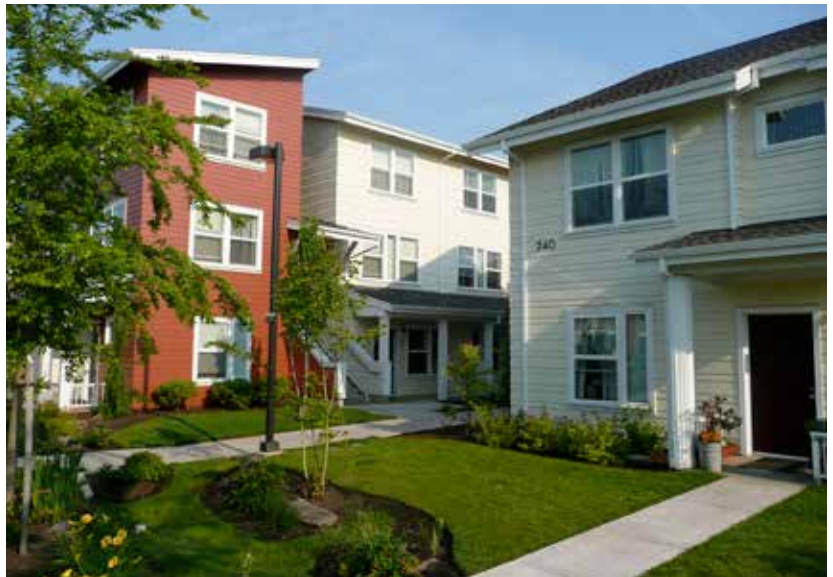
Fig. A.6.S3: Internal landscaping provides trees and other vegetation sized to create an attractive, mature site.
