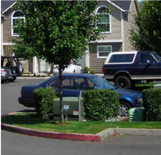
Fig. B.4.S3: Ground level utilities are placed in landscape islands screened by evergreen shrubs.
