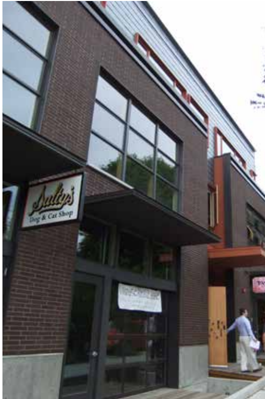
Fig. B.6.S1.b: The variety of materials, primarily brick which contrasted with concrete and metals, creates interest and texture on the facade.
