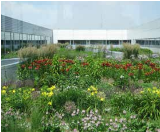
Fig. B.4.S10.a: A vegetated roof surface contributes to the reduction of energy usage and improves on-site stormwater treatment.
