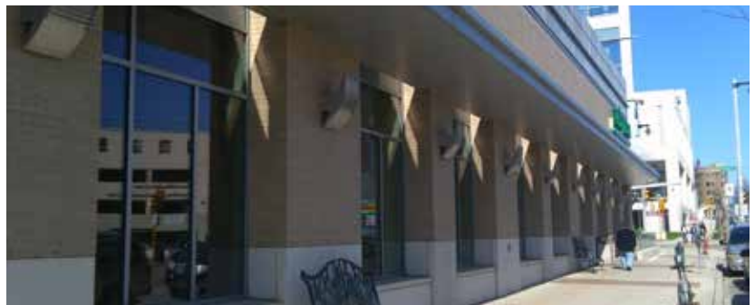
Fig. B.4.S6: A combination of projections/recesses and changes in wall plane are used to establish depth.
