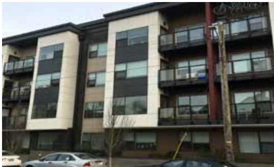
Fig. A.5.S4: Outdoor private space is provided in the form of balconies attached to each unit.
