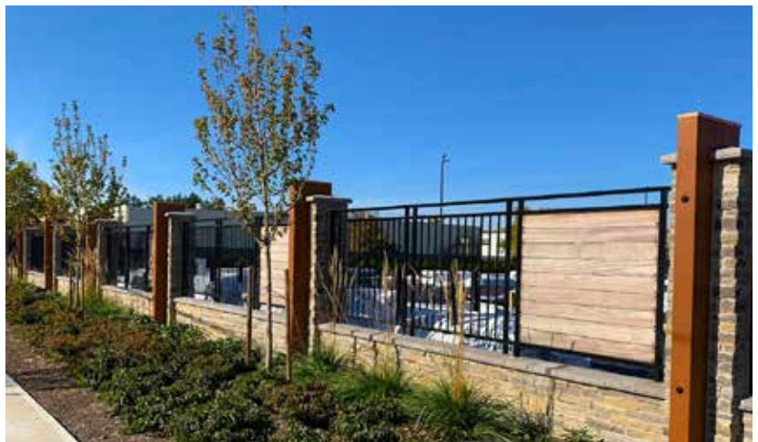
Fig. A.6.S2: Site trees are provided along the front yard setback, supported by stakes at time of planting.
