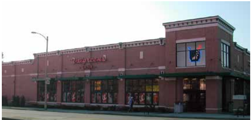
Fig. B.4.S7: Projecting facade elements, including solar shades and wall sconces are present along street facing facades.
