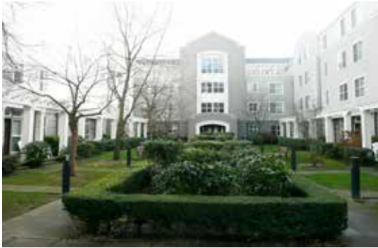
Fig. A.5.S3. A well-maintained courtyard shared open space at the center of a multifamily development.
