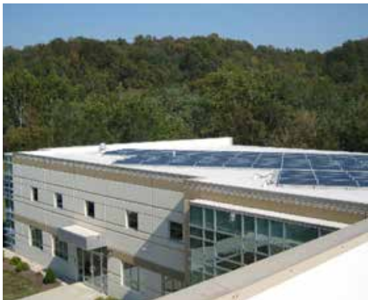
Fig. B.4.S4.a: Solar arrays on top of an industrial building.
