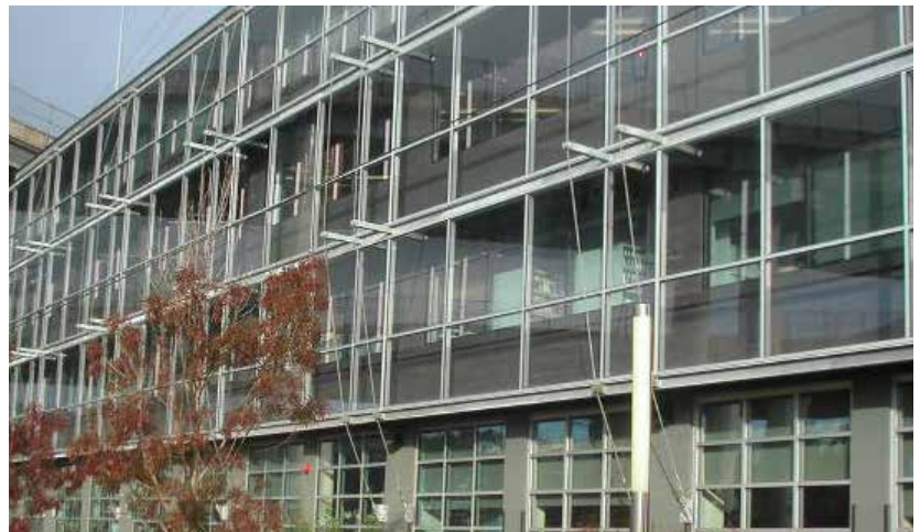
Fig. B.4.S4.b: A high level of transparency located on the south facing building facade takes advantage of passive solar collection.
