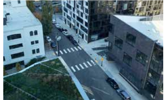
Fig. B.2: Low-sloped roofs utilize landscaped roof systems and white roofs with a high Solar Reflectance Index to reduce the heat island effect.
