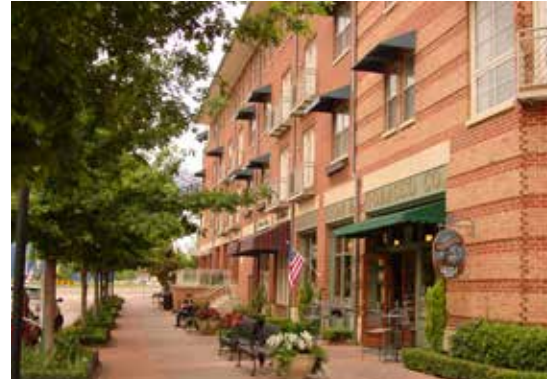
Fig. B.6: Multiple finishes of brick and stone are used together to establish texture in the facade.
