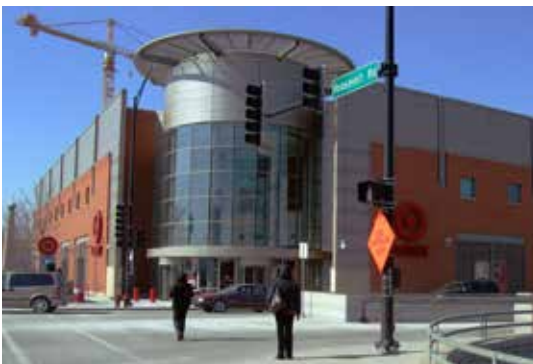
Fig. B.3.S2 and S3: A large commercial building utilizing a corner entry to provide access from both streets and a visible change in form from adjacent facade sections.
