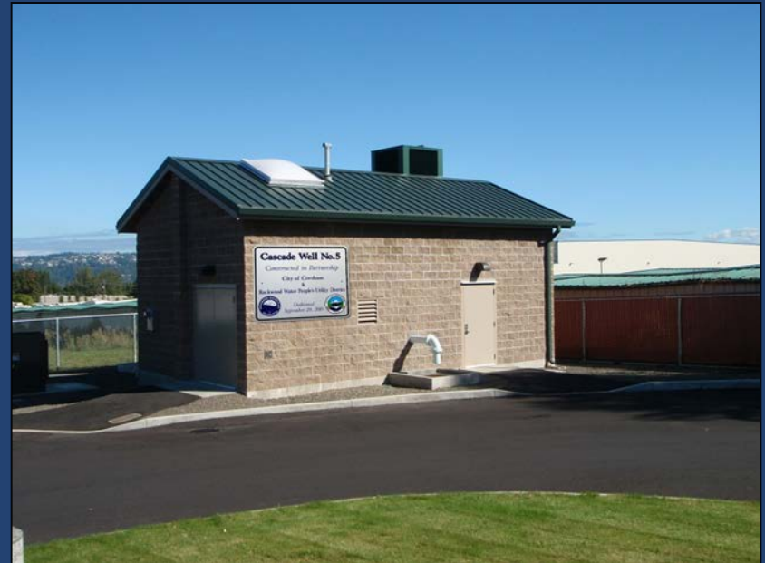
Cascade No. 5 Well House Supplemental source since 2010 Partnership Between City of Gresham and Rockwood Water People's Utility District
