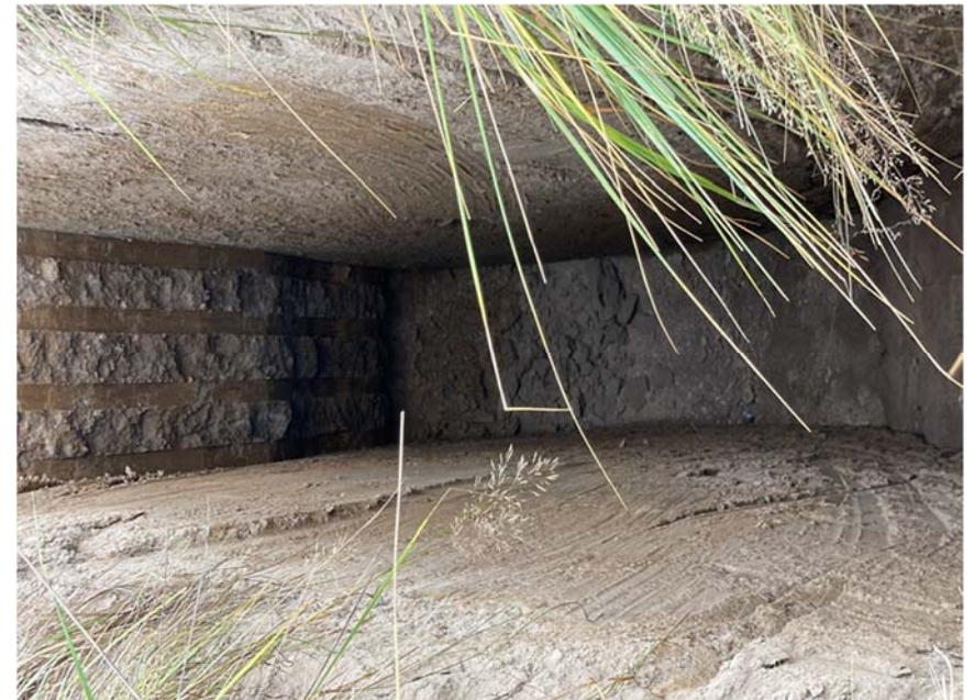
Photo J. View of Geotech test pit on August 4, 2023 documenting no groundwater table within 17 feet below surface.
