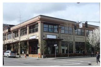
Fig B.2.d.4: A building which is designed with pilasters and belt courses to enhance the facades.
