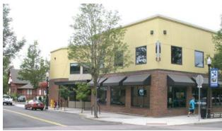
Fig B.3.d.4 (2): A building base that utilizes a change in material.
