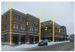
Fig B.1.d.1: A building with a large footprint is divided into multiple masses, each greater than 25% of the footprint.
