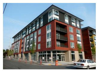
Fig. B.2.d.7: In DCC, buildings should establish base, middle and top.
