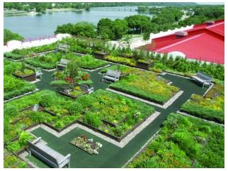
Fig A.6.c.1 and 2: A modular vegetated roof system reduces stormwater and insulates the roof surface.
