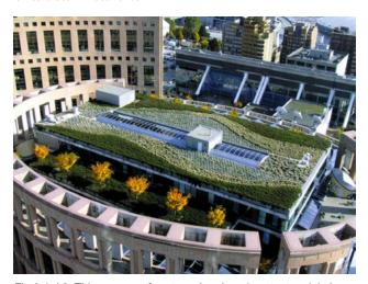
Fig A.6.d.2: This green roof system absorbs rainwater to minimize stormwater run-off and provides opportunity for possible water re-use.
