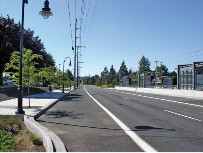
View of pedestrian-friendly development on E. Burnside Street west of SE 187th Avenue in Rockwood.
