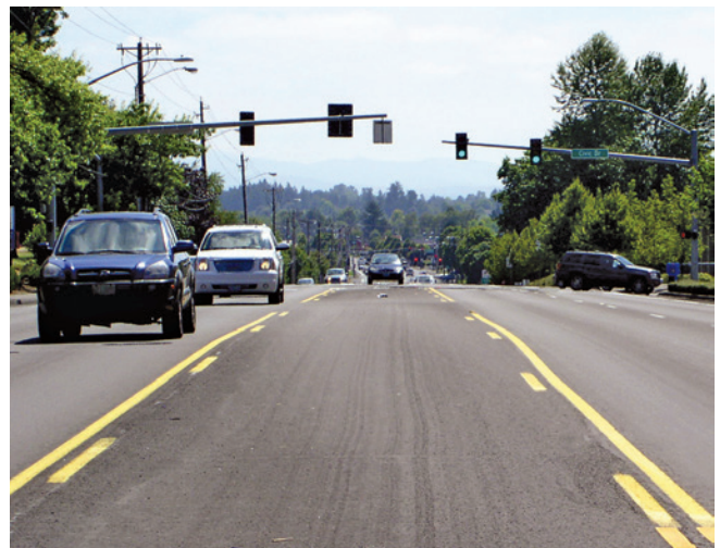
Signals at the NE Burnside Road/Civic Drive.
