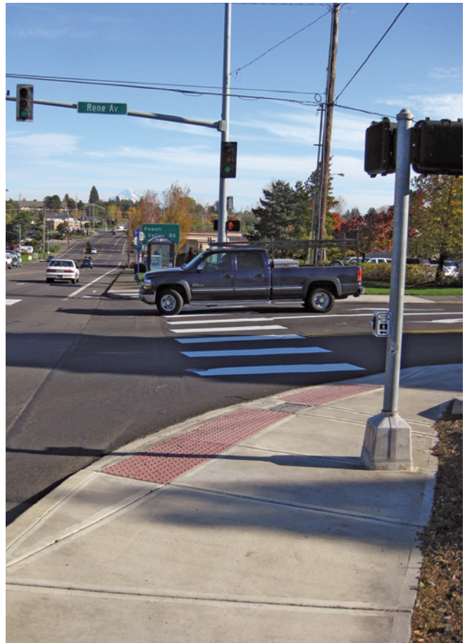
An ADA-compliant curb ramp on SE Rene Avenue.
