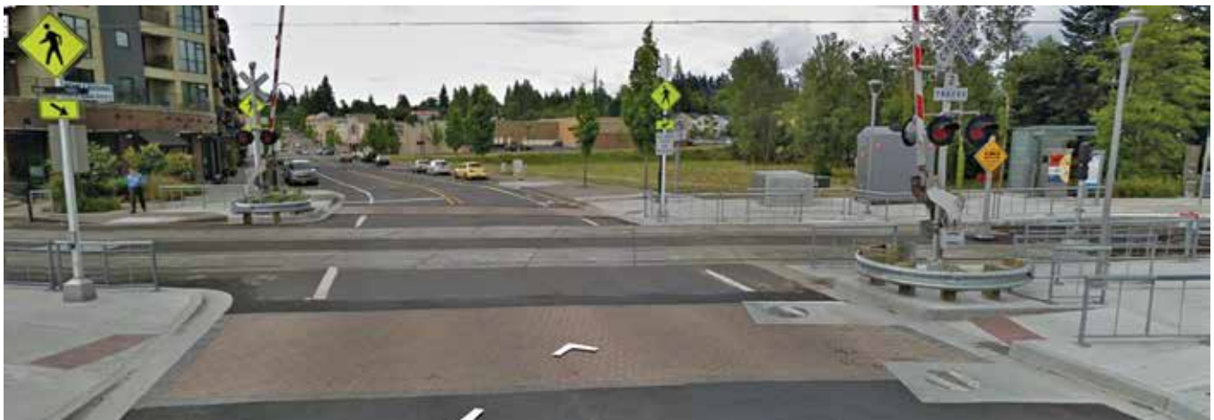
A pedestrian crossing created with a paver design in Gresham's Civic Neighborhood.
