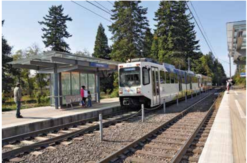
The Civic Drive MAX station serves the pedestrian district in the Gresham Regional Center.
