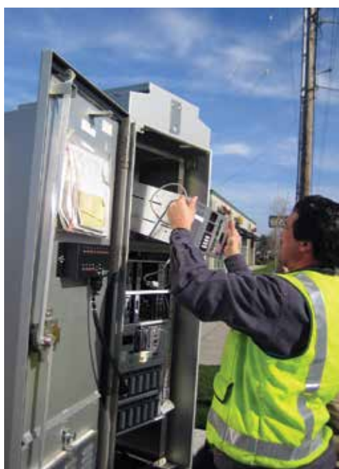
City of Gresham electrician Tony Sepich adjusts the traffic light signals.
