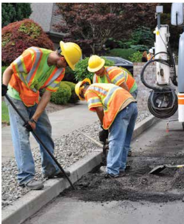
City Transportation Operations crews repair a street's pavement.
