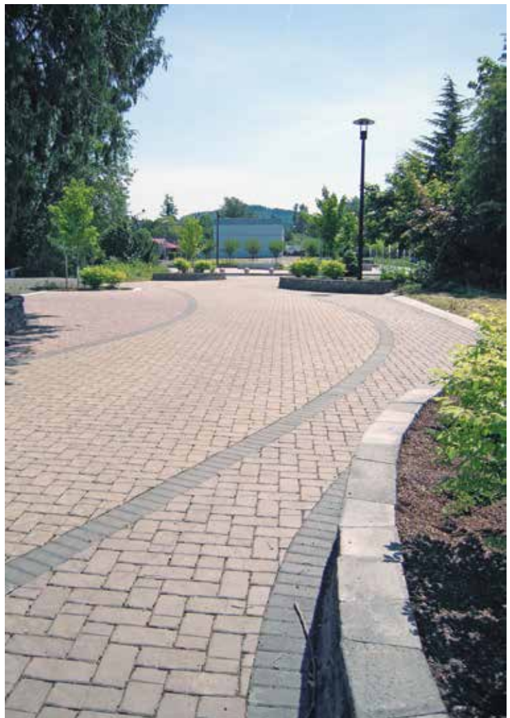
Beech Street captures stormwater runoff and filters soil pollutants.
