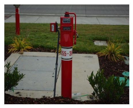
Appendix III Page 1 of 2 Approved Standard Hydrant Assembly with Storz Adapter Installed
