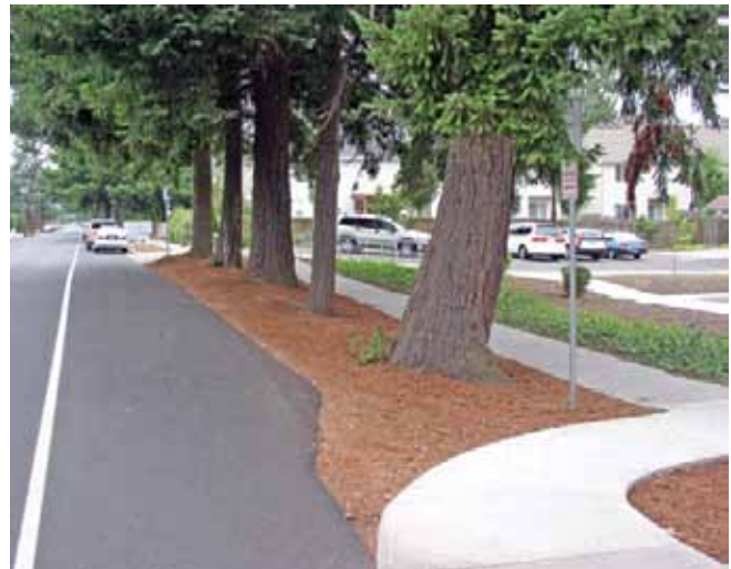
Gresham’s award-winning Yamhill Green Street project diverted sidewalks around existing trees.
