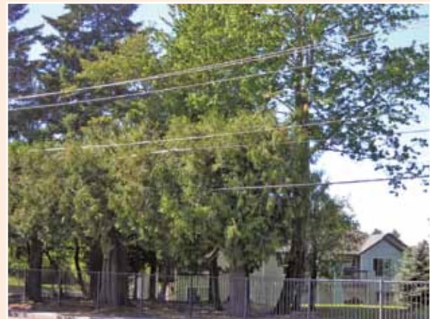
Tree and power line conflicts.
