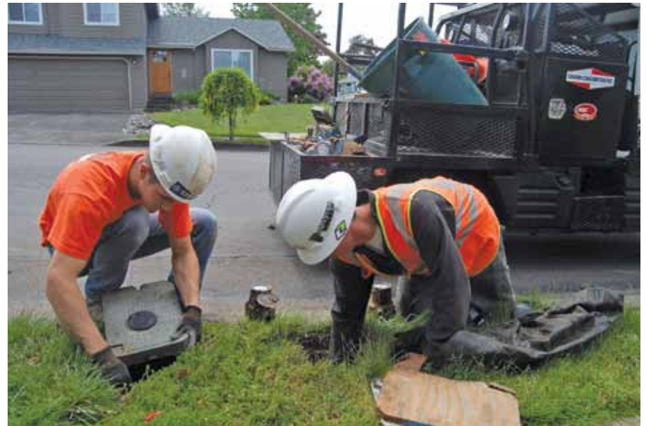
Technicians installed residential "smart" water meters in 2010.
