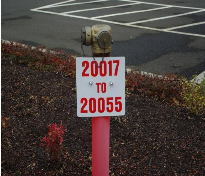
Example 2: Flexible metal sign with address range of buildings served. Includes pad locked PIV handle.
